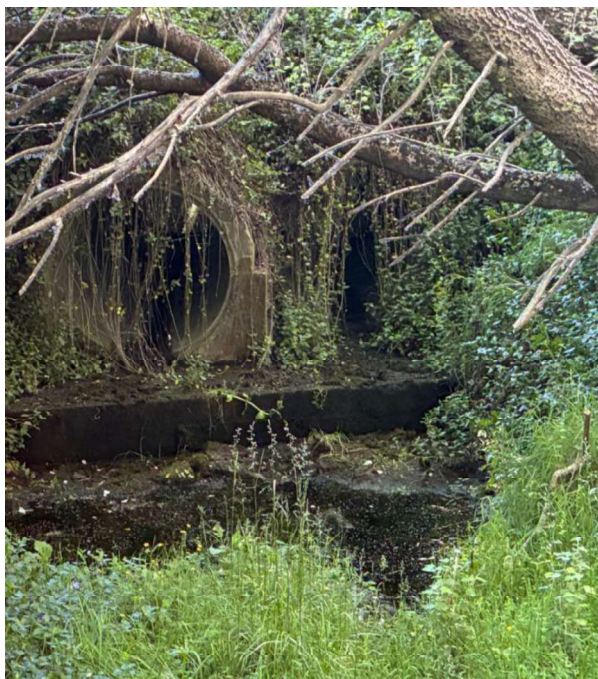
Figure 32: Existing twin culvert on SH2 – view looking from downstream to upstream
