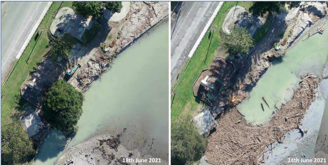
Figure Sixty Nine. Comparison between the Tokomaru Reserve and playground drone orthomapping dated 18 th June and 24 th of June 2021. Note the removed tree, the overhanging concrete pad bottom left and the erosion at the turn around bay.
