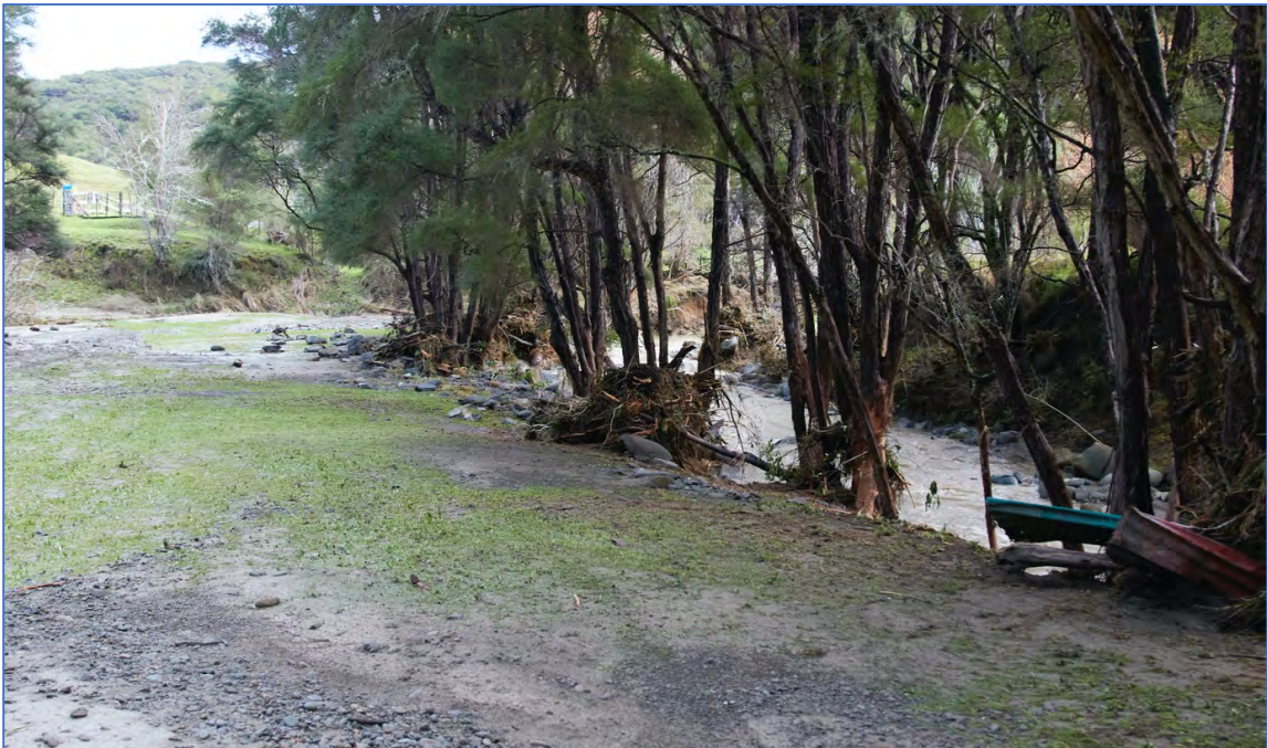
Figure Thirty Eight. Photograph upstream of the ford on Kaiawha Road showing debris caught up in the trees and mud deposited across the valley floor.
