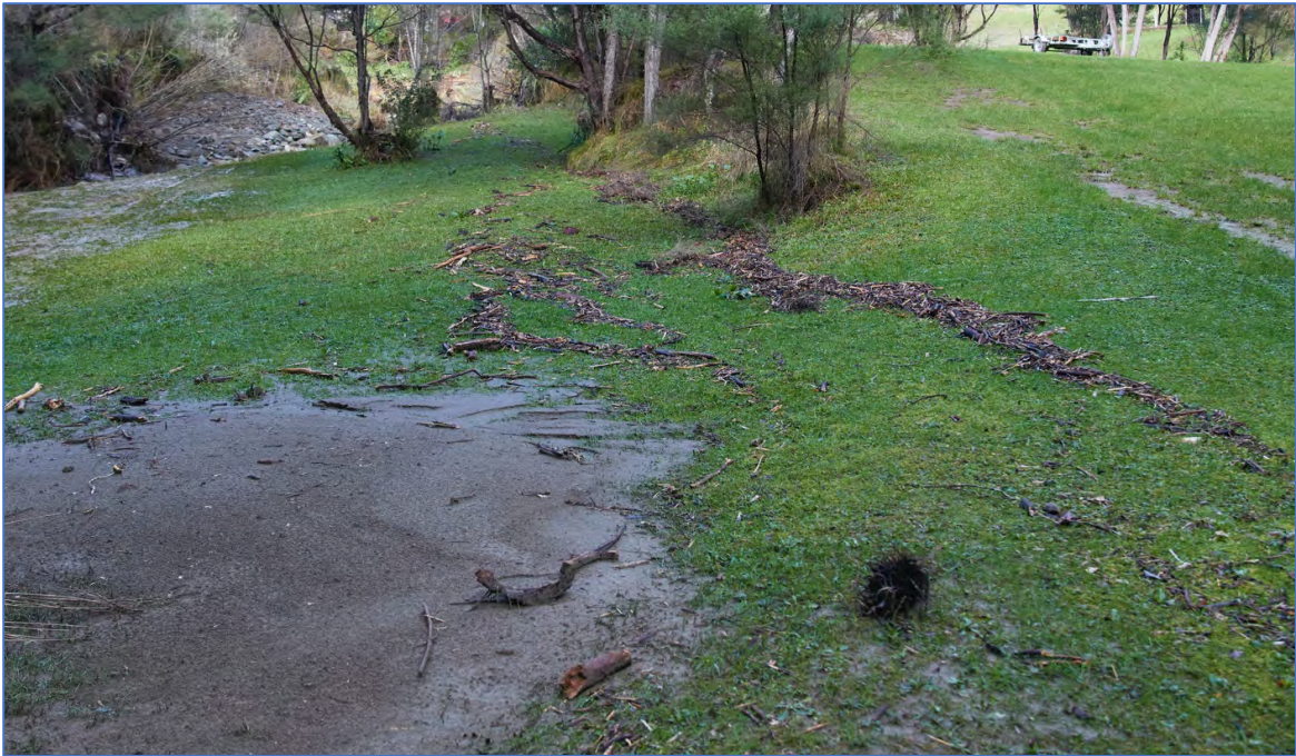
Figure Thirty Nine. Photograph upstream of the ford on Kaiawha Road showing the edge of the flood spread against higher ground.
