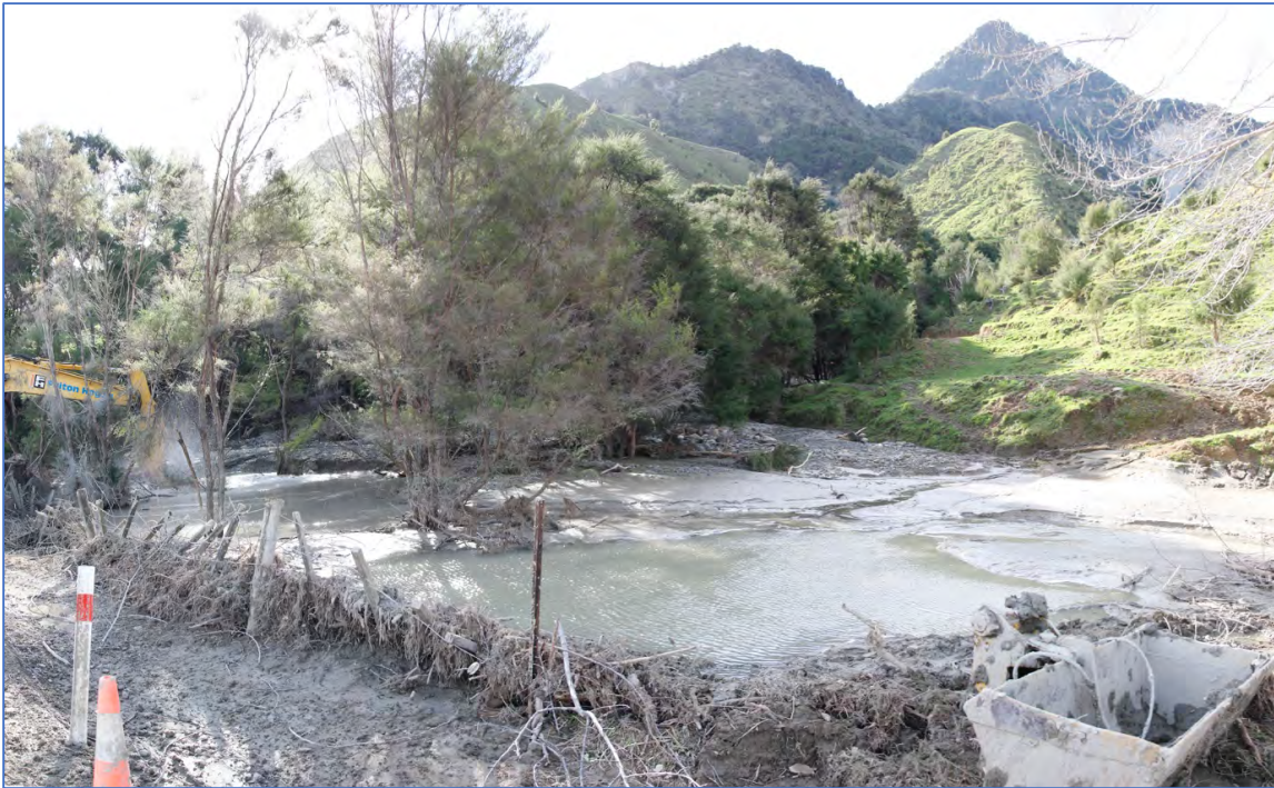
Figure Fifty Two. View of culvert on State Highway 35 north of Tokomaru Bay prior to clearing. Note the extensive infill of debris and the indications of overtopping on the fenceline.
