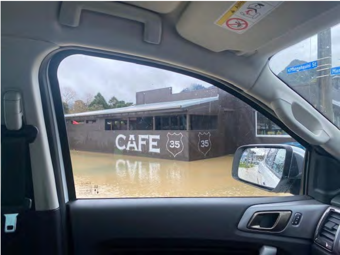
Figure Forty Seven. Flooding at café 35, Tokomaru Bay. It is assessment that the flooding here was the result of overland flow rather than flooding from the Mangahauini River.
