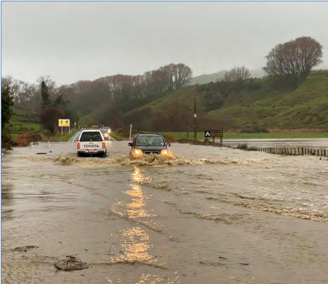
Figure Fourteen. Flooding on State Highway 35 south of Tolaga Bay.
