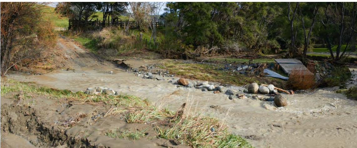
Figure Thirty Six. Photograph of the ford 650m upstream of the bridge on State Highway 35 showing the depth of silt deposition (bottom left), the height of the flood spread based on the debris layer and the mobilised boulders on the ford path.
