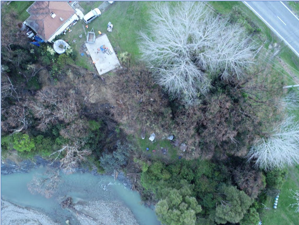
Figure Twelve. Drone footage of property at Hiruharama, south of Ruatoria where slipping from a side creek is threatening a house.
