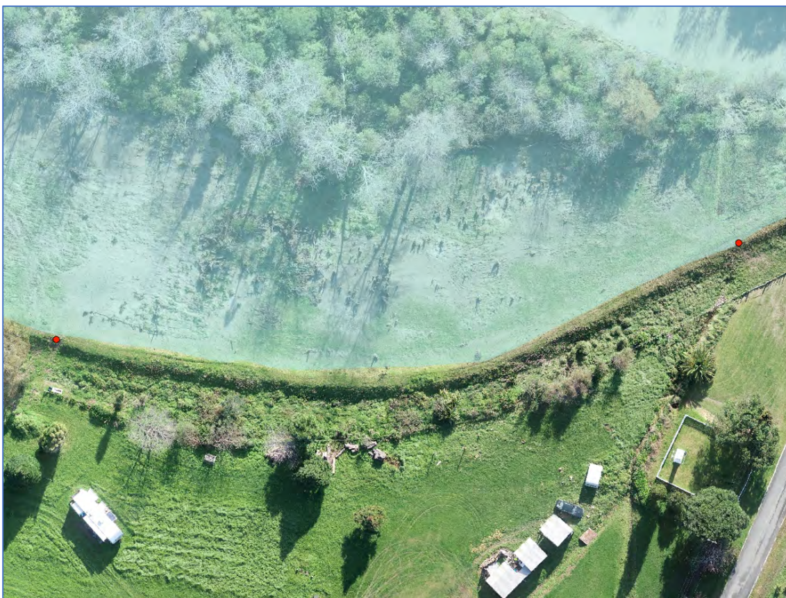
Figure Fifty Six. View of the lower true right bank of the Mangahauini showing the two overtopping points. The old road is shown at far right.
