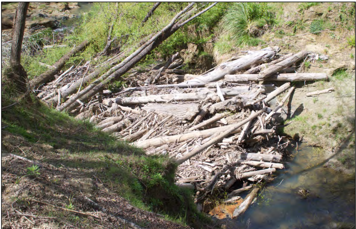
Figure Two. View of the logjam comprising pine logs and slash, and showing the collapsed willows.
