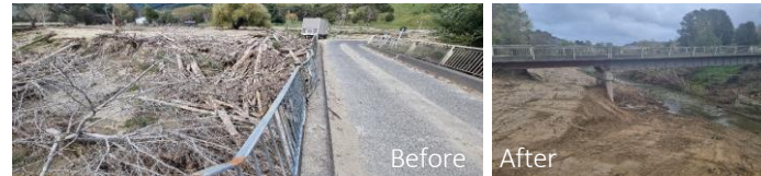
Frasers Bridge Kanakanaia Road Debris Removal
