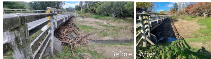
Christopher Bridge Wharekopae Road Debris Removal
