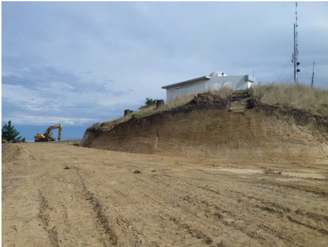
Figure 10: Eastern cut slope below observatory shortly after completion in 2015.
