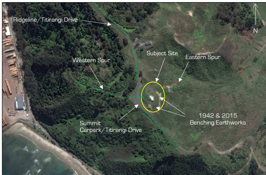
Figure 2: Subject site (circled in yellow) and surrounding land [source: Tairawhiti Maps].
