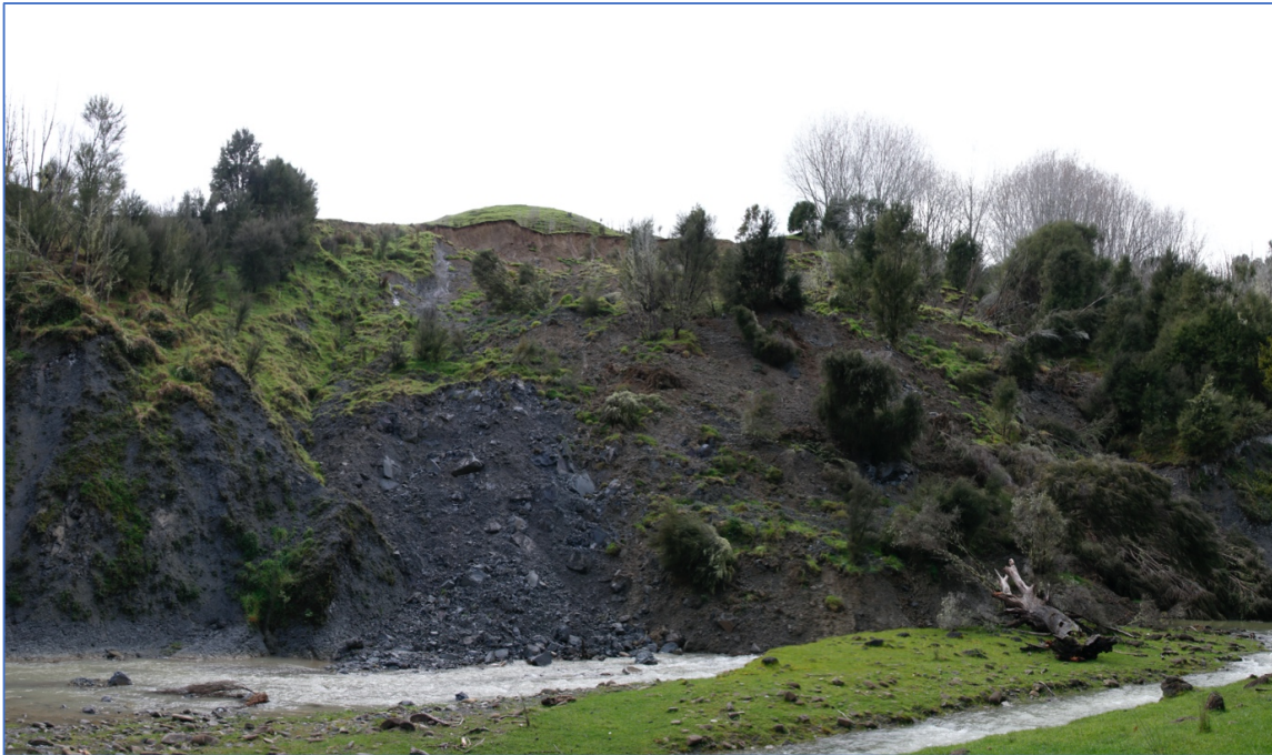
Figure Two. View of the landslide showing the area affected and the large headscarp at the top of the failure. The main channel is flowing against the toe of the slope while the secondary channel that normally accommodates flood flow is now taking some of the flow as a result of the partial damming of the river. This secondary channel was enlarged on the same day to release the water dammed up behind the slip.
