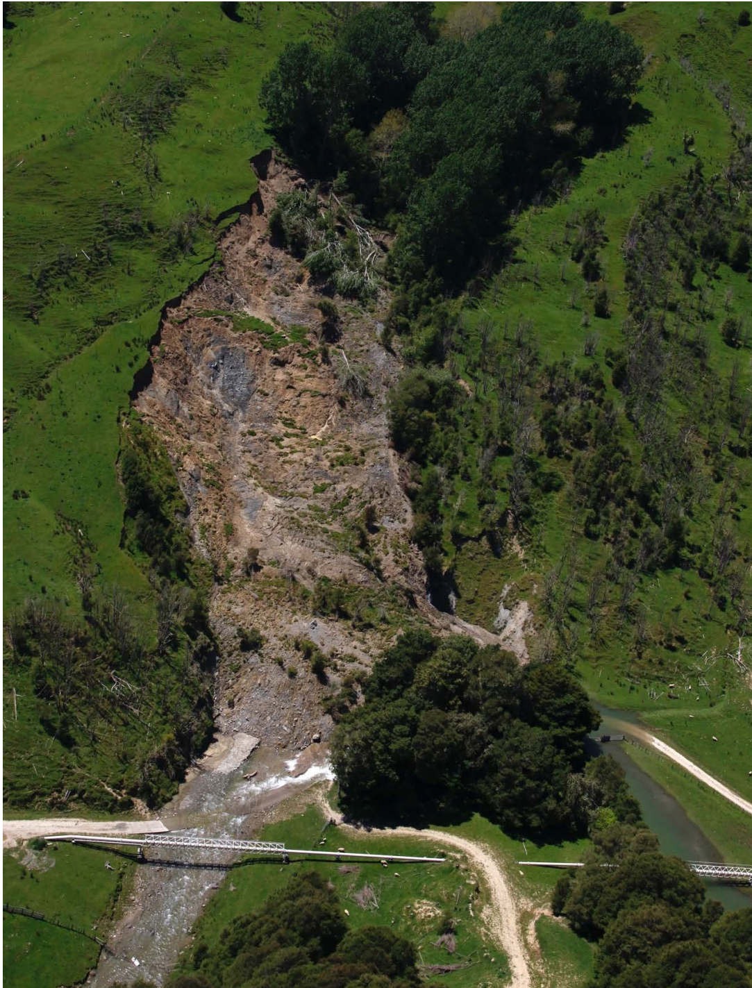
Figure Ten. View of the landslide after the November storm. The proposed bridge would be located at the bottom left of this image.
