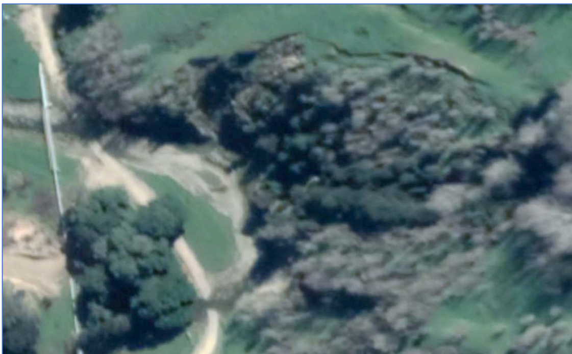
Figure One. October 15 th 2019 satellite image of the landslide area showing the obvious tension crack. Also note that the river is cutting into the toe of the slope.
