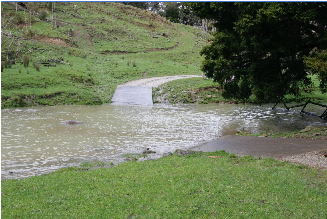
Figure Three. View of the ford immediately upstream showing the increase in water depth over the ford, prior to the channel being enlarged to reduce water levels.
