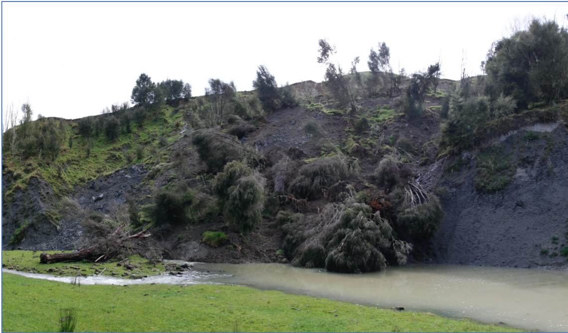
Figure Four. View of the slip from upstream showing the ponding and the water being diverted into the flood channel
