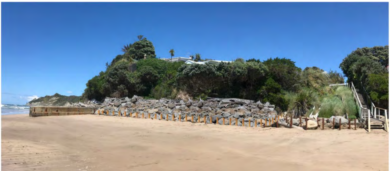
Figure 15: Photo from Viewpoint 12, looking southwest from near the water's edge at the existing situation towards the face of the rock revetment, to where it abuts the groyne. NB: this is a photo merge of two photos. A3 size version of the viewpoint is provided in Appendix D .
