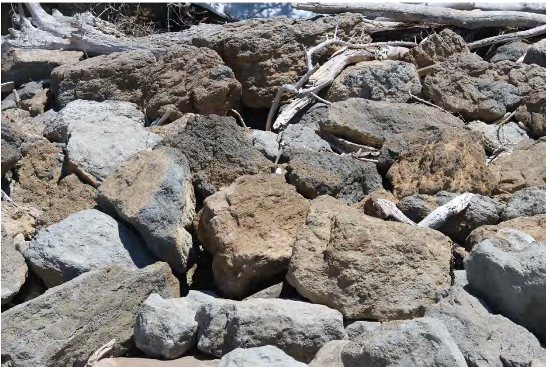
Figure 5 - Image of existing rock revetment extending from the south side of the groyne. This local weathered limestone rock mix type is proposed for the new rock revetment fill. Due to natural ocean processes, the proposed rock revetment will also naturally accumulate driftwood, which will help visually integrate the rock revetment into the coastal environment.
