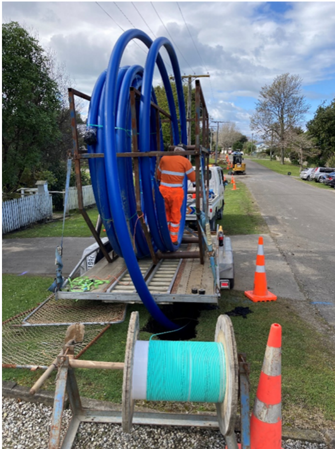
125mm PE water pipe being drawn along Walsh Street after drilling.
