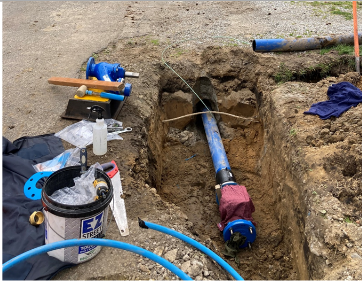
Installing Fire Hydrant Walsh Street
