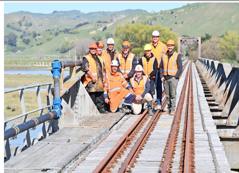
Muriwai water main crossing Rail Bridge
