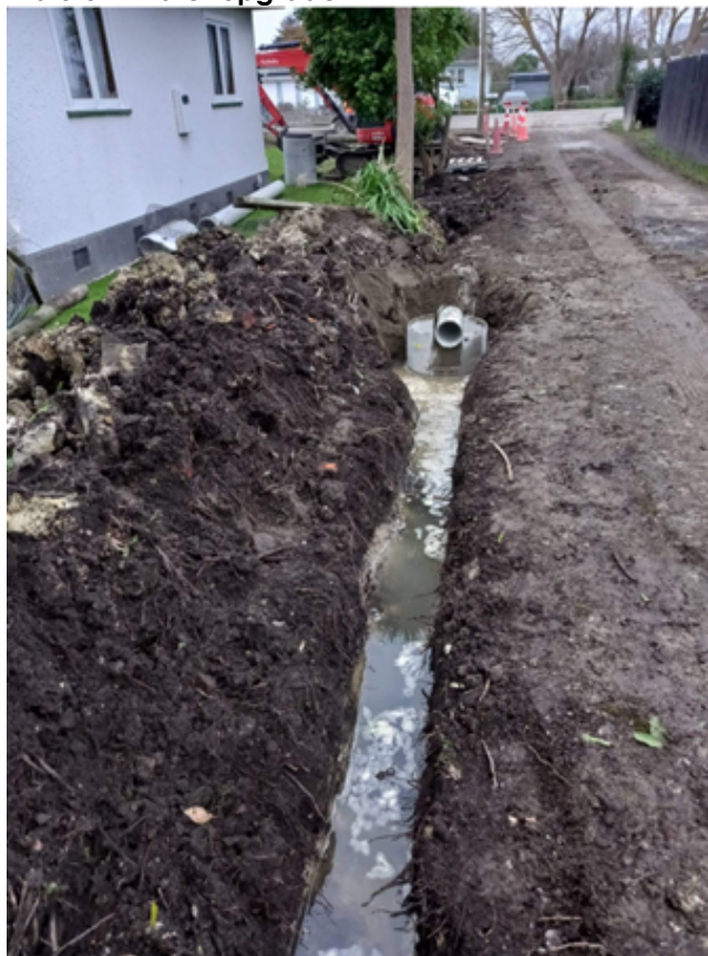
Slow progress due to ongoing wet weather
