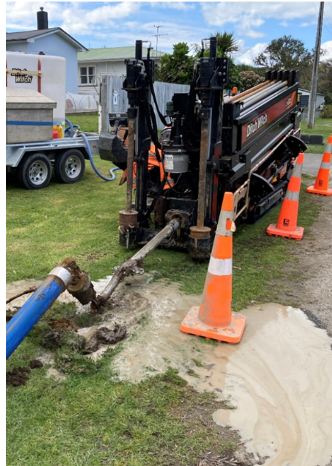
Directional drilling to replace water main
