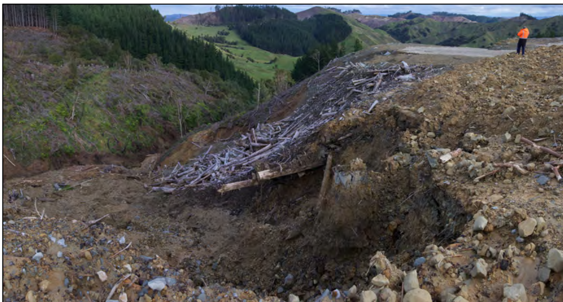
Figure Thirty Eight. View looking west to the harvest residues at Landing 11 showing the slash supported by corduroy logs. Also visible is the trimline for the debris flow from the site. This may have been a retaining wall of logs that has failed.
