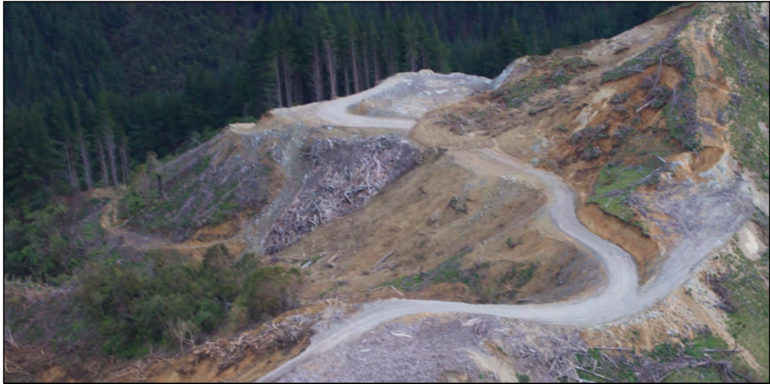
Figure Thirty Nine. View of Landing 11 (with Landing 9 at the bottom of the image and Landing 10 at far right) showing the failure from the top of the slope (top right) crossing the road. The edge of the debris apron for this event does not appear to have extended beyond the birds-nest but may have triggered a slope failure at the edge of the birds-nest.
