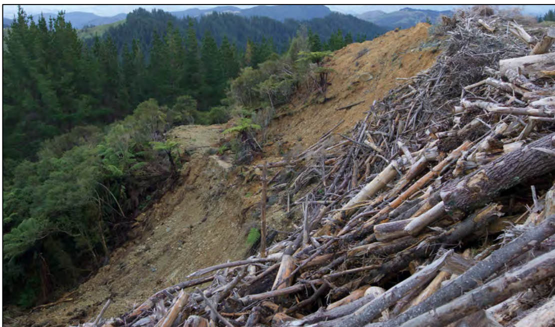
Figure Twenty Five. View of the south western side of Landing 8 looking west showing a failed bench in the middle ground and the slash apron extending down slope to the south.
