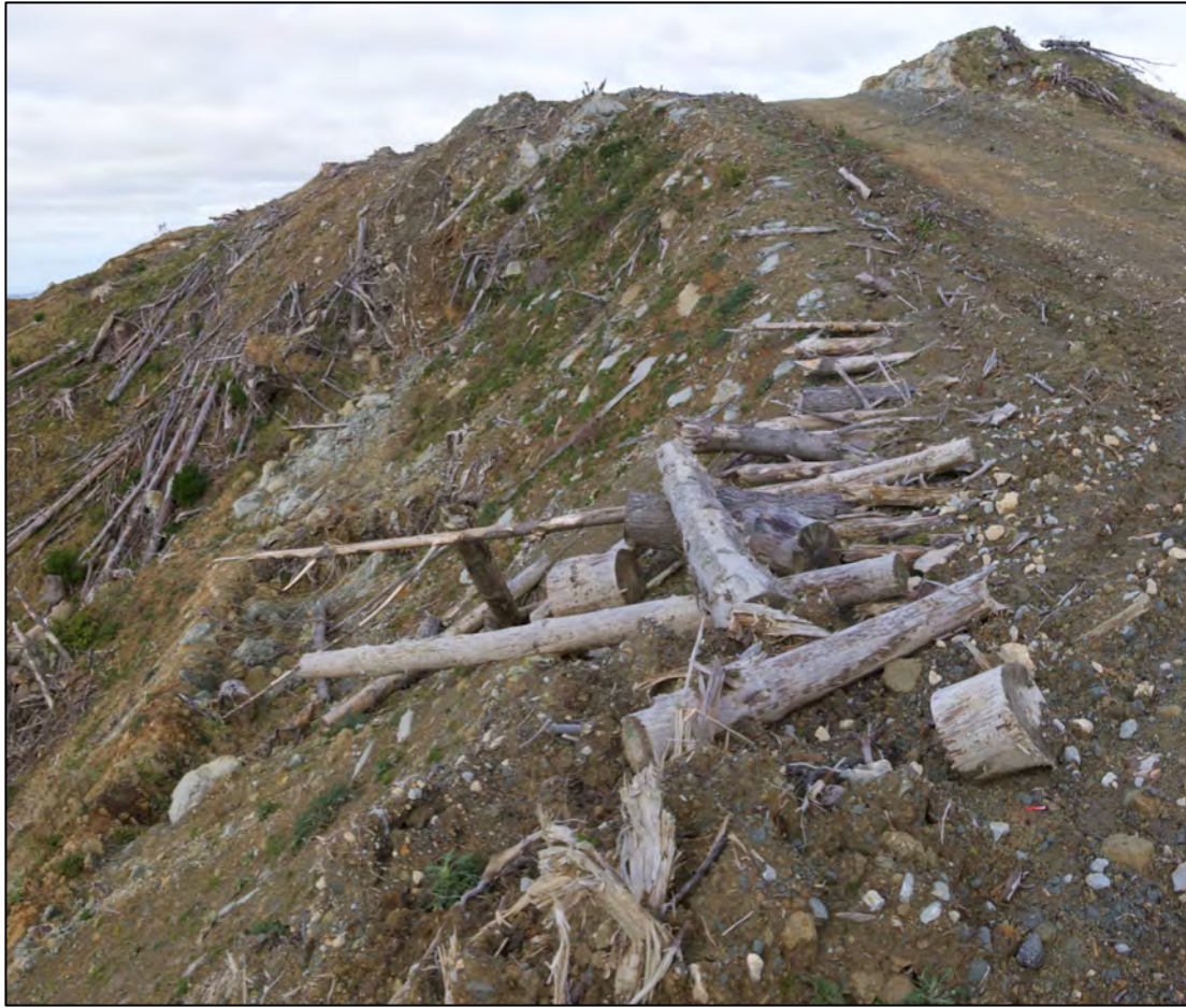
Figure Twenty. Use of corduroy west of Landing 6 (in background). Use of such corduroy is not an effective long term means of supporting the roadway and in this instance a log has been driven into the fill slope below in an attempt to improve support but this has started to rotate downslope. Note the present of slovens mixed up with the corduroy. The loss of harvest residues downslope at Landing 6 is evident in the background.
