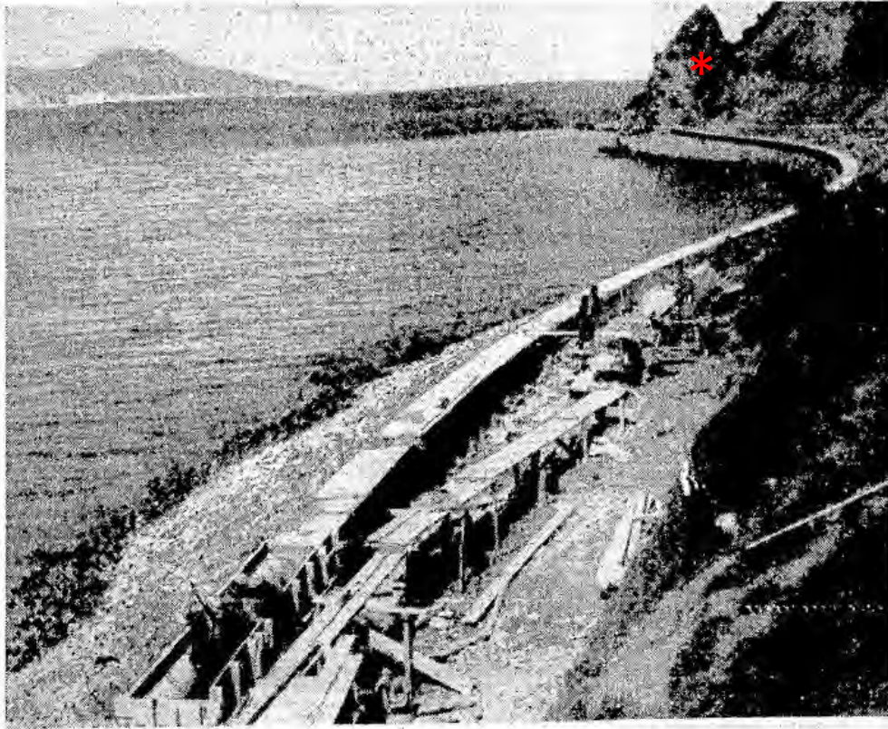
Building a sea-wall on the route of the East Coast railway, the construction of which is nearing completion. This wall, in the neighbourhood of Waikokopu, is to protect the new line from erosion along a shingly beach, where the sea constantly alters the coastline.
