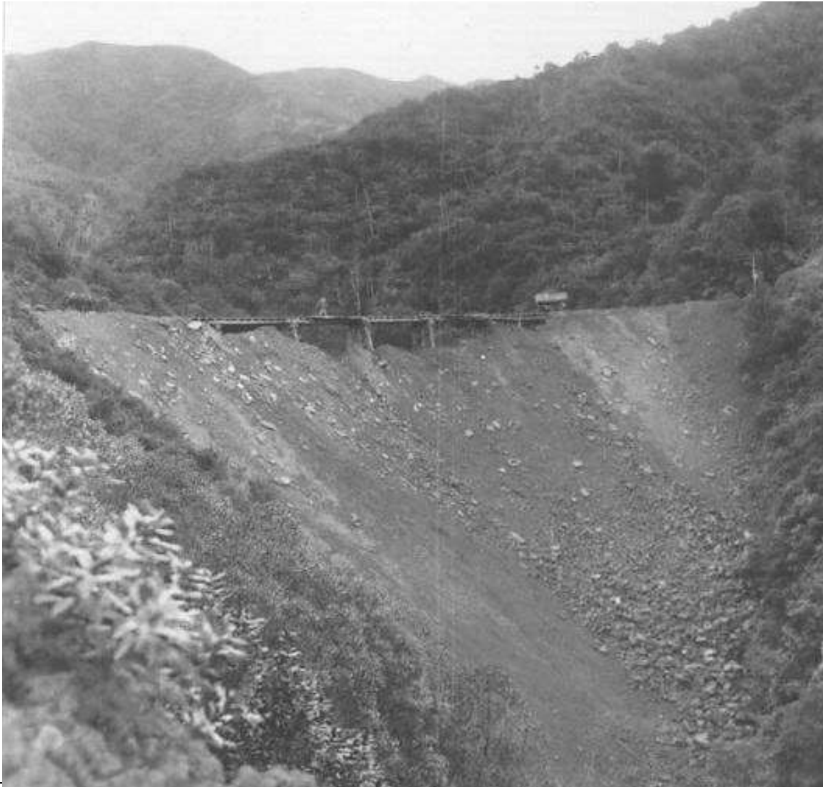
1936 historical photo during Wharekakaho Tunnel 26 construction – tunnel spoil was railed out over gully and then either bottom or side tipped to form unconsolidated embankment. Note photo is also good indication of typical excavated rockmass materials in other embankments and fills in Beach Loop and Kopuawhara Valley areas.
