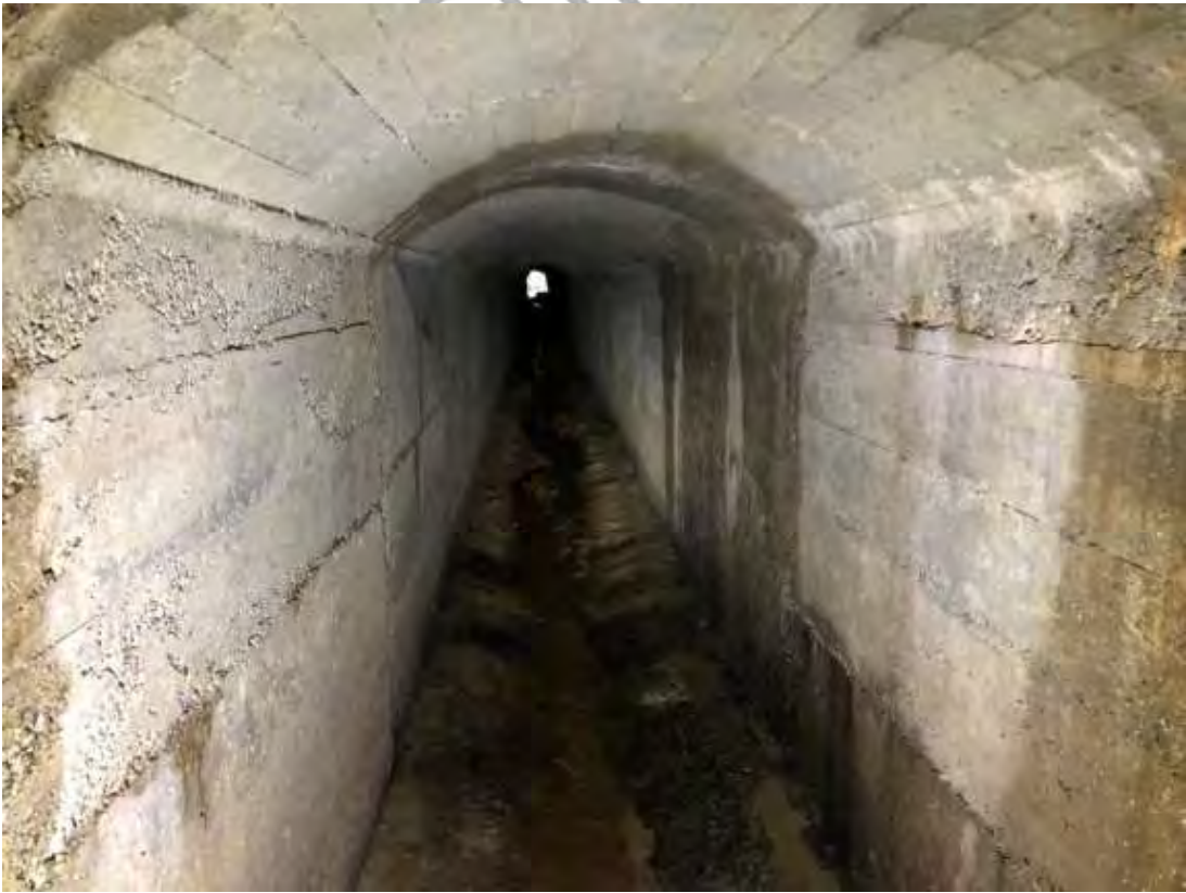
Drainage drive photos – above is nominal 2.5*2.5 tunnel section for 60m downstream of arch culvert
