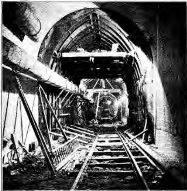
WAIKOURA TUNNEL, NORTH END. VIEW SHOWING STAGES OF CONSTRUCTION: TIMBERING IN BACKGROUND; STEEL FORMWORK IN MIDDLE DISTANCE; AND FINISHED LINED TUNNEL IN FOREGROUND.
