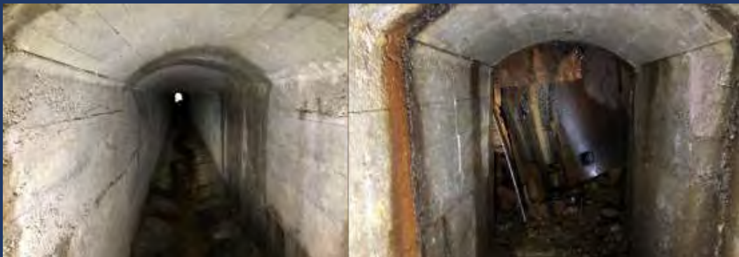
Example of blocked culvert at inlet side
