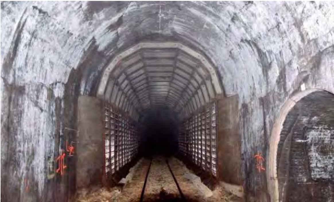
Photo showing lining support at approx. track meterage 359.4km (TBC). Track has also been lowered to allow passage for high cube containers at this location.
