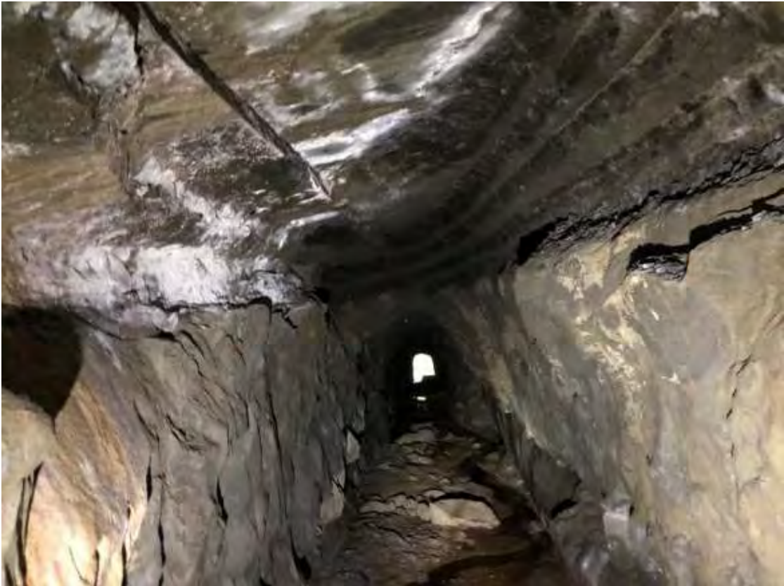
Drainage drive photos – above is nominal 2.5*2.5 tunnel section for 60m downstream of arch culvert
