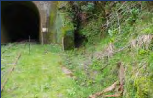
Blocked swale drainage and culvert inlet outside Tunnel 23
