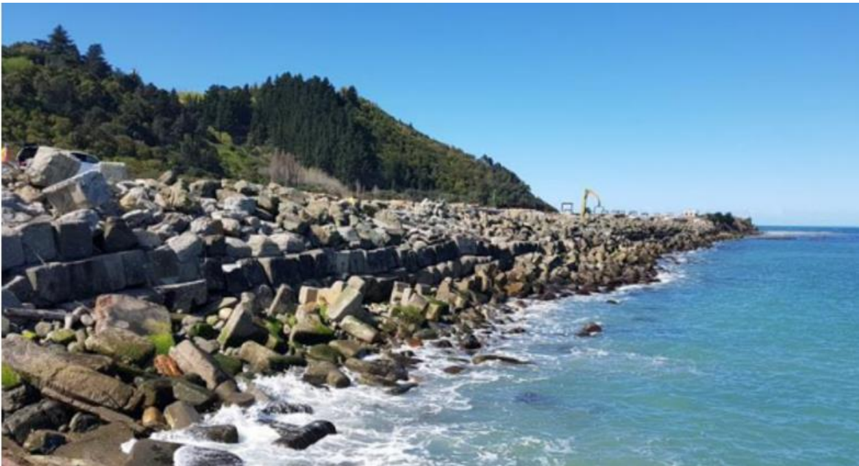
Figure 56: Photograph of Southern Logyard Revetment Wall that will be partially removed
