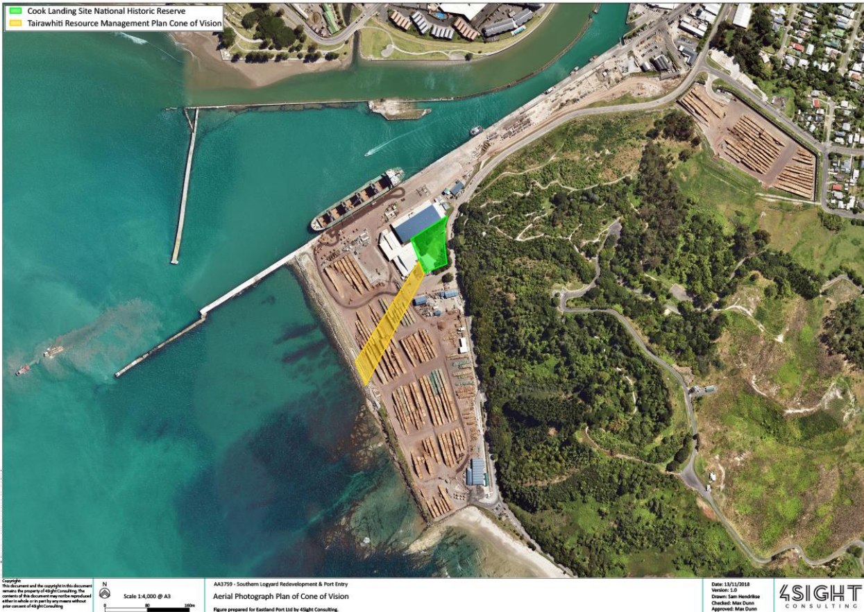
Figure 92: Port Aerial Photograph with Cone of Vision
