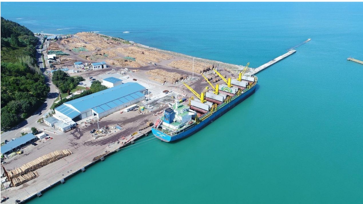
Figure 17: Oblique Aerial Photograph of Wharf 8
