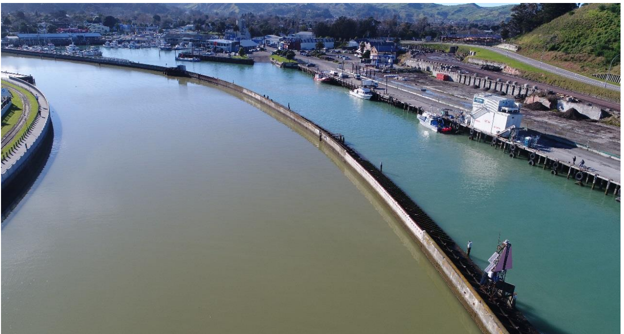
Figure 31: Drone Photograph of Turanganui River Flood Tide
