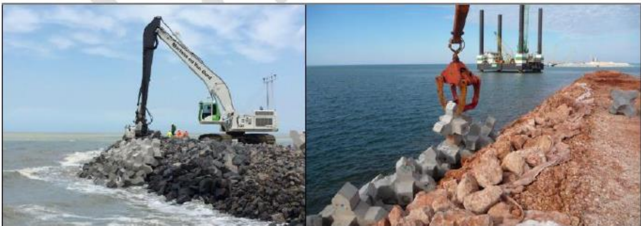
Figure 61: Photographs of Concrete from Similar Reclamation Projects
