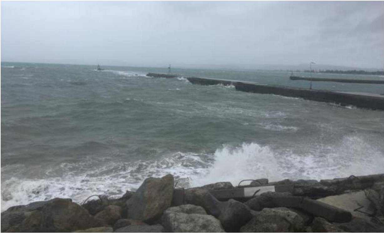
Figure 22: Photograph of Largely Submerged Outer Breakwater
