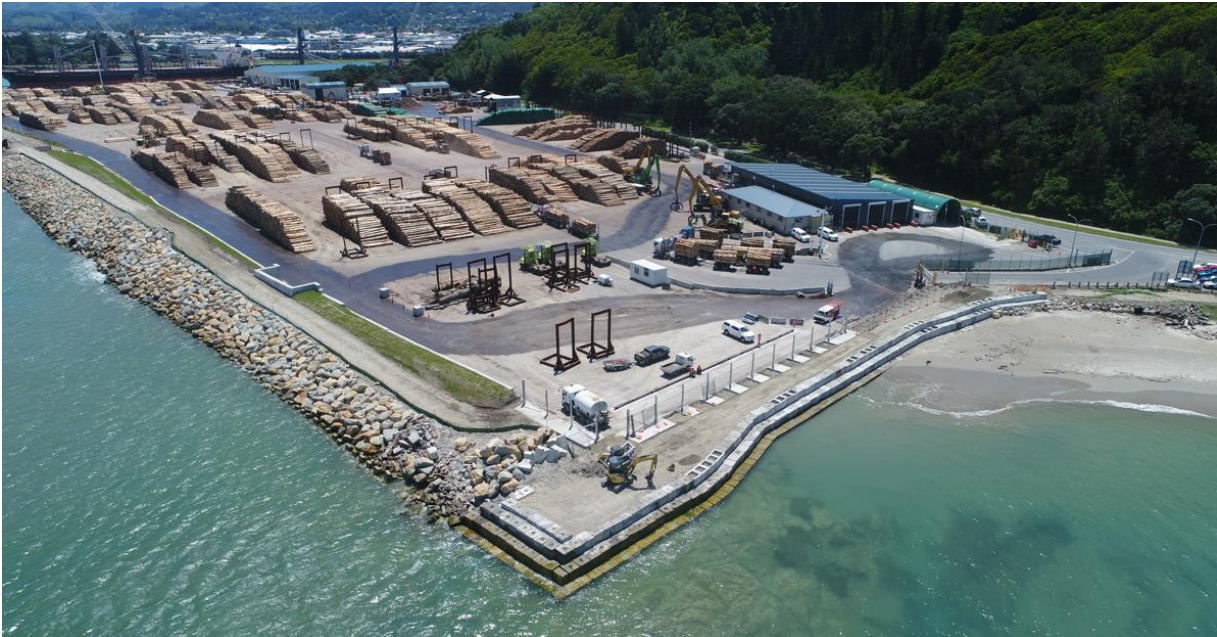
Figure 49: Southern Logyard Seawall maintenance and Waikahua Seawall Upgrade works completed to April 2022
