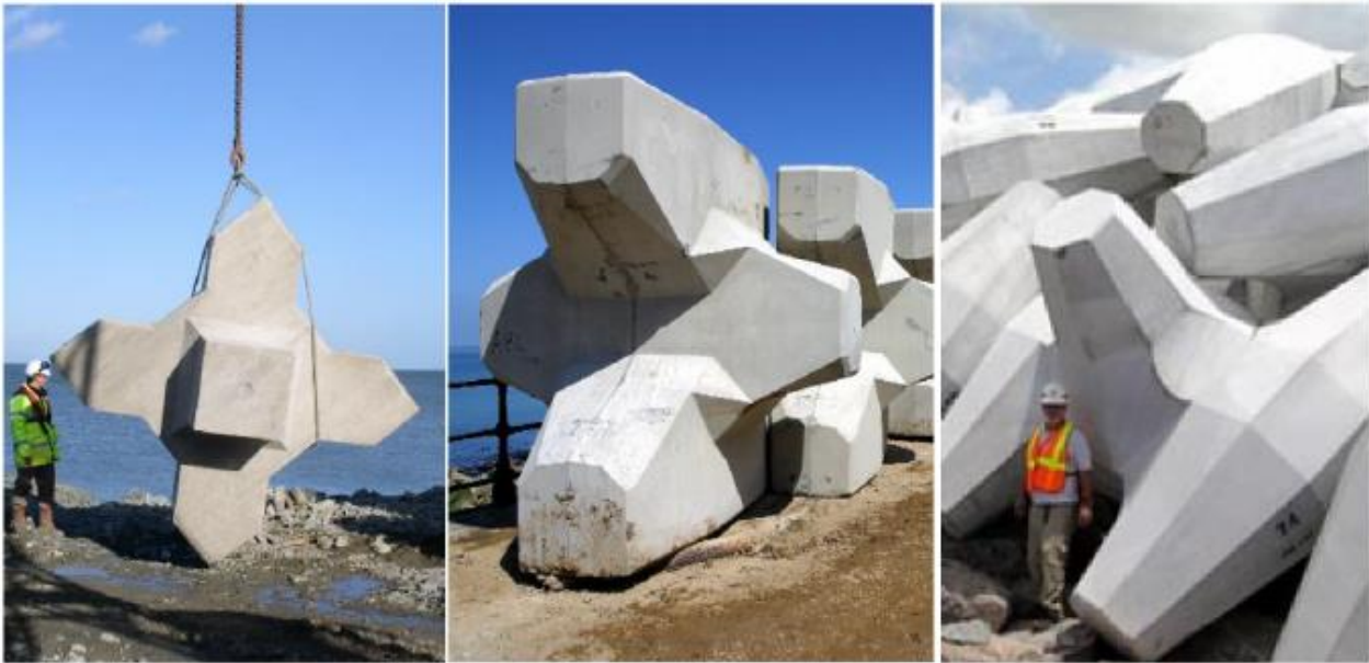
Figure 60: Photographs of Concrete Armour Units Expected to be Used on the Proposed Reclamation
