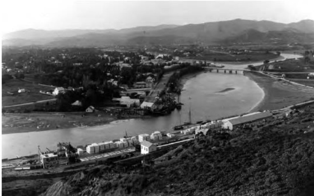
Figure 6.3 – Reclamation of mudflats: 1891 vs 1909 a
