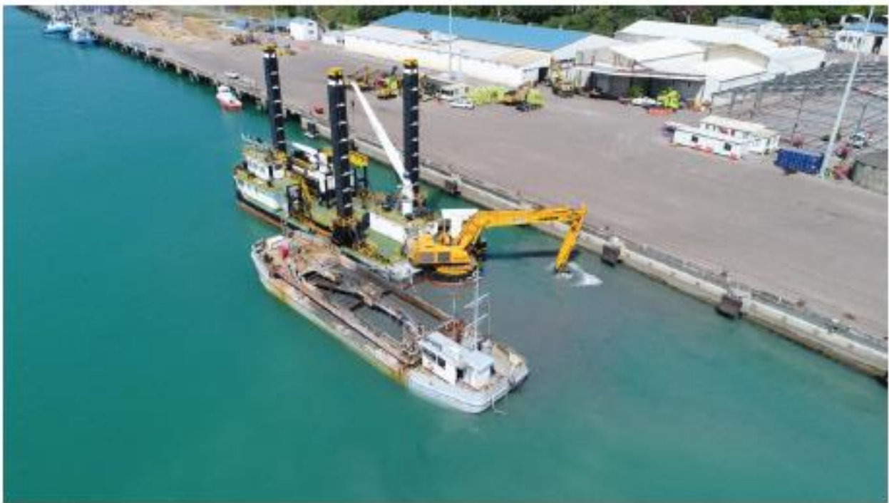
Figure 82: Photograph of Backhoe Dredging Operation at Gisborne Port
