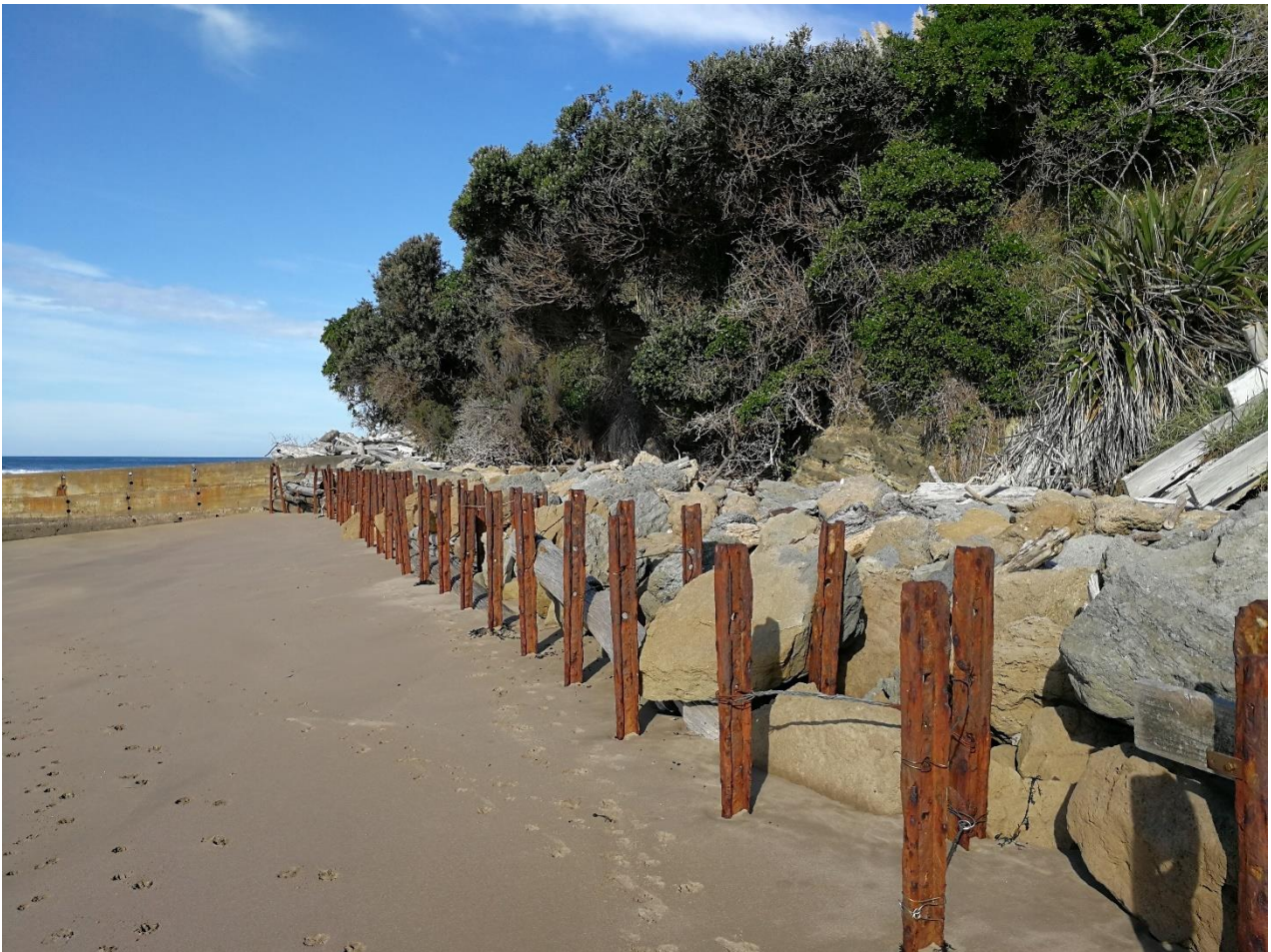
Figure 9: Photo of existing seawall, facing south towards concrete groyne (Source: 4Sight)
