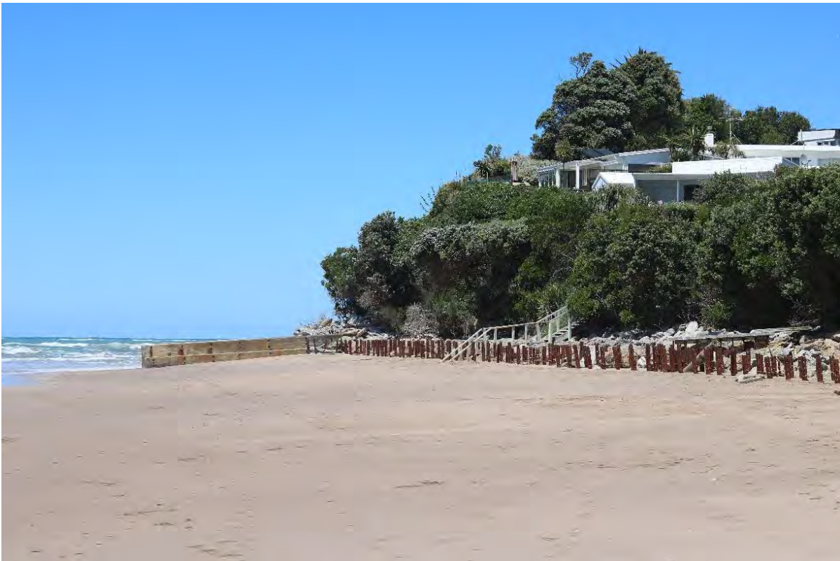
Figure 17: Photo from Viewpoint 13, 100m away from the site, looking southwest along the beach as the rock revetment starts to recede into the wider view. A3 version is provided in Appendix D .
