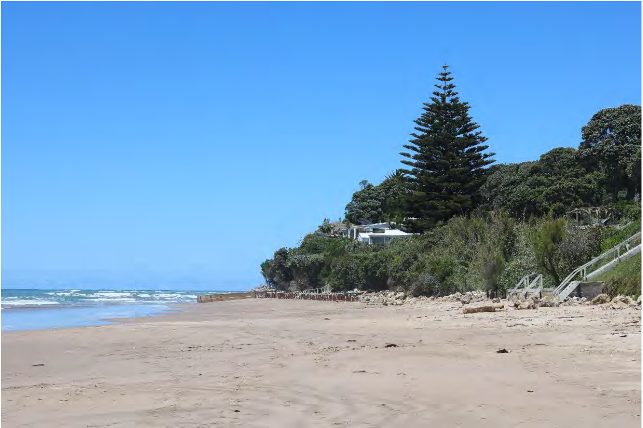
Figure 18: Photo from Viewpoint 14, 145m away from the site, looking southwest along the beach as the rock revetment starts to recede into the wider view. A3 version is provided in Appendix D .
