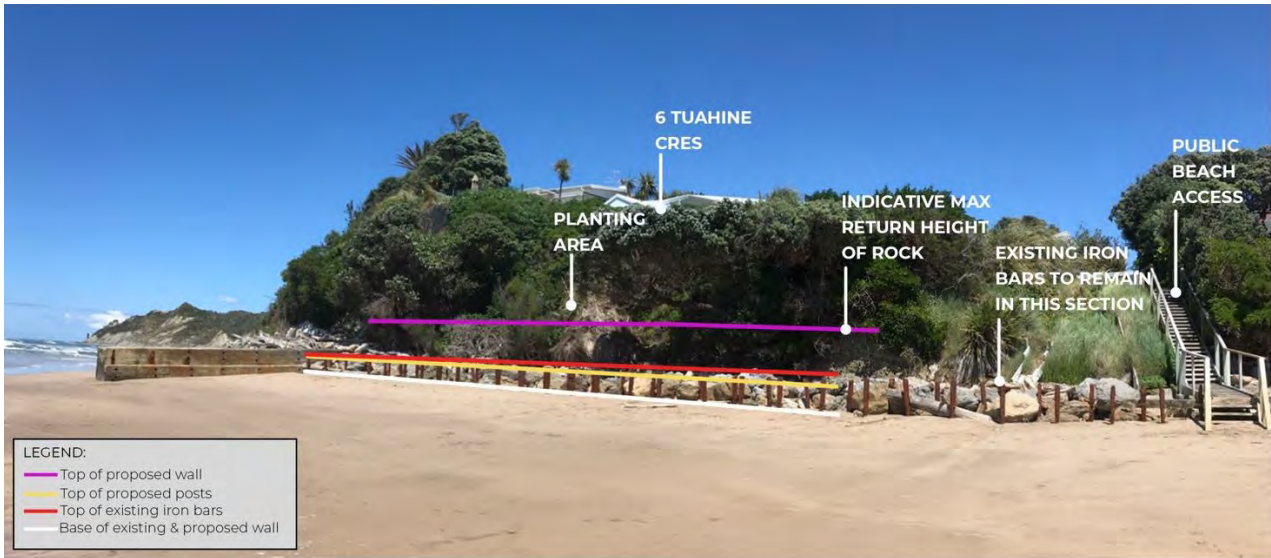
Figure 14: Photo from Viewpoint 12, looking southwest from near the water's edge at the existing situation towards the face of the rock revetment, to where it abuts the groyne. NB: this is a photo merge of two photos. A3 size version of the viewpoint is provided in Appendix D .
