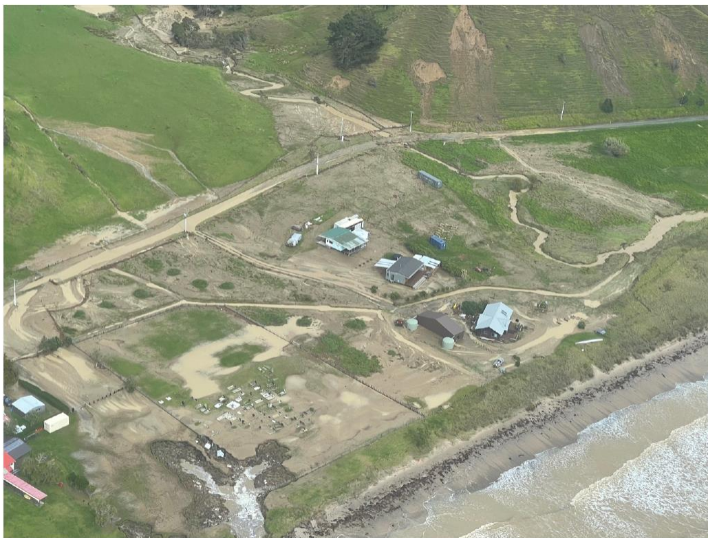
Figure 5.9: Aerial photo of Lockwood Road, the Hawaii Stream and urupa erosion at the south end of Anaura Bay (source GDC)
