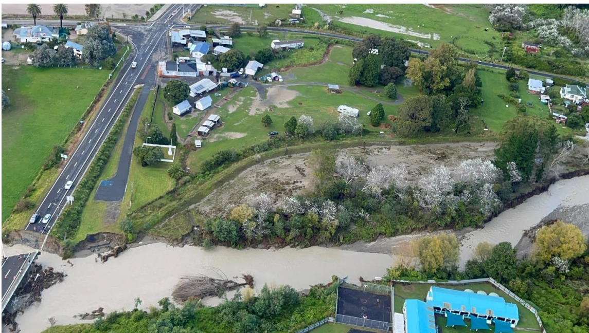
Figure 5.6: Mangahauini River SH35 bridge washout, with the stopbank on the true right bank (Photo source GDC).
