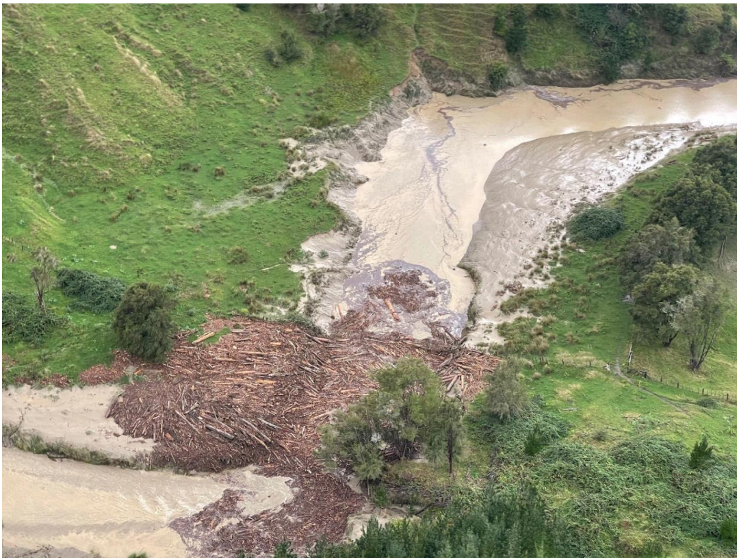
Figure 5.3: Photo of wood debris on the Waitoroko Stream showing the river damming impact of large amounts of wood debris.
