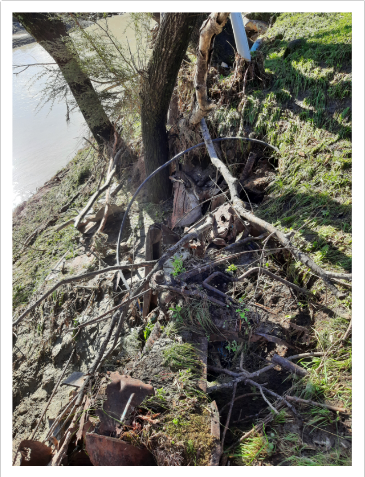
Metal protruding from the Tokomaru Legacy Landfill after the 19 JUN 21 flood event.
