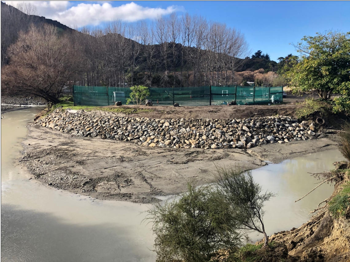
Figure 1: Rock revetment protection sealing the landfill in August 2020. Source: GDC.
