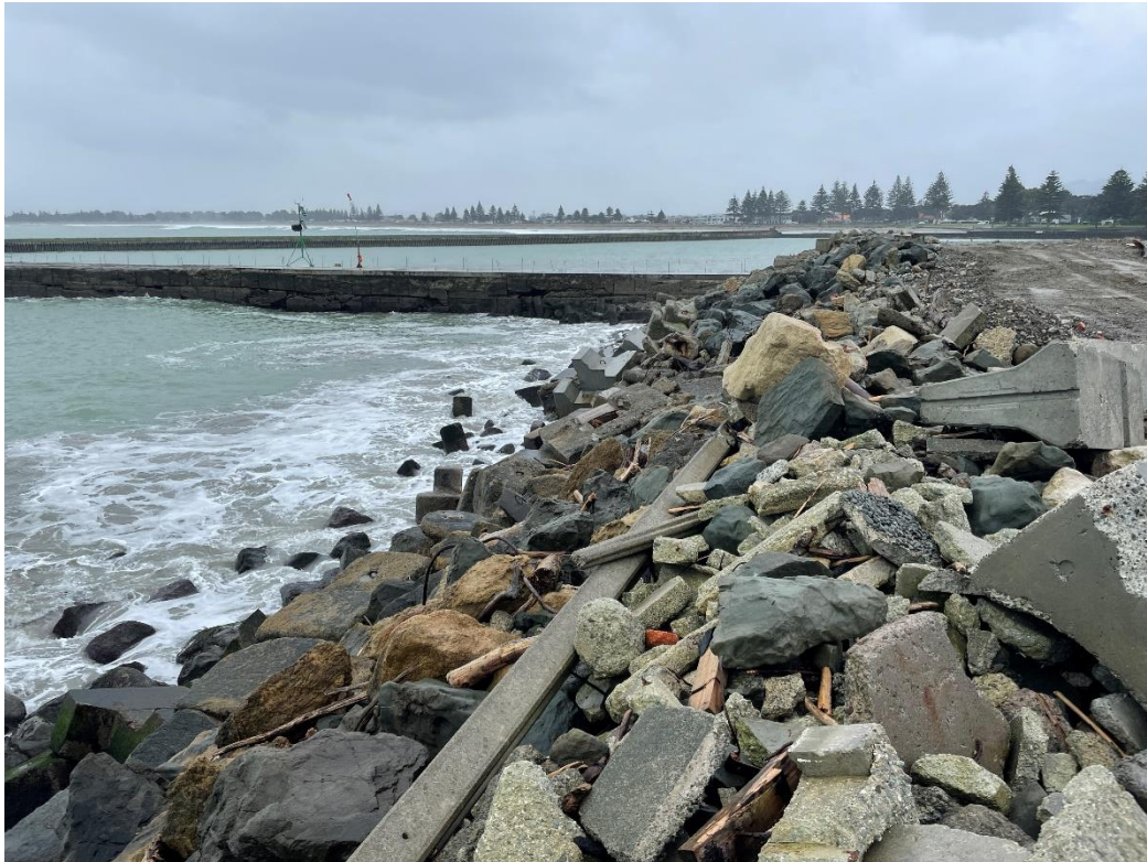
Figure 7: Outer seawall dominated by large rocks and concrete pieces.
