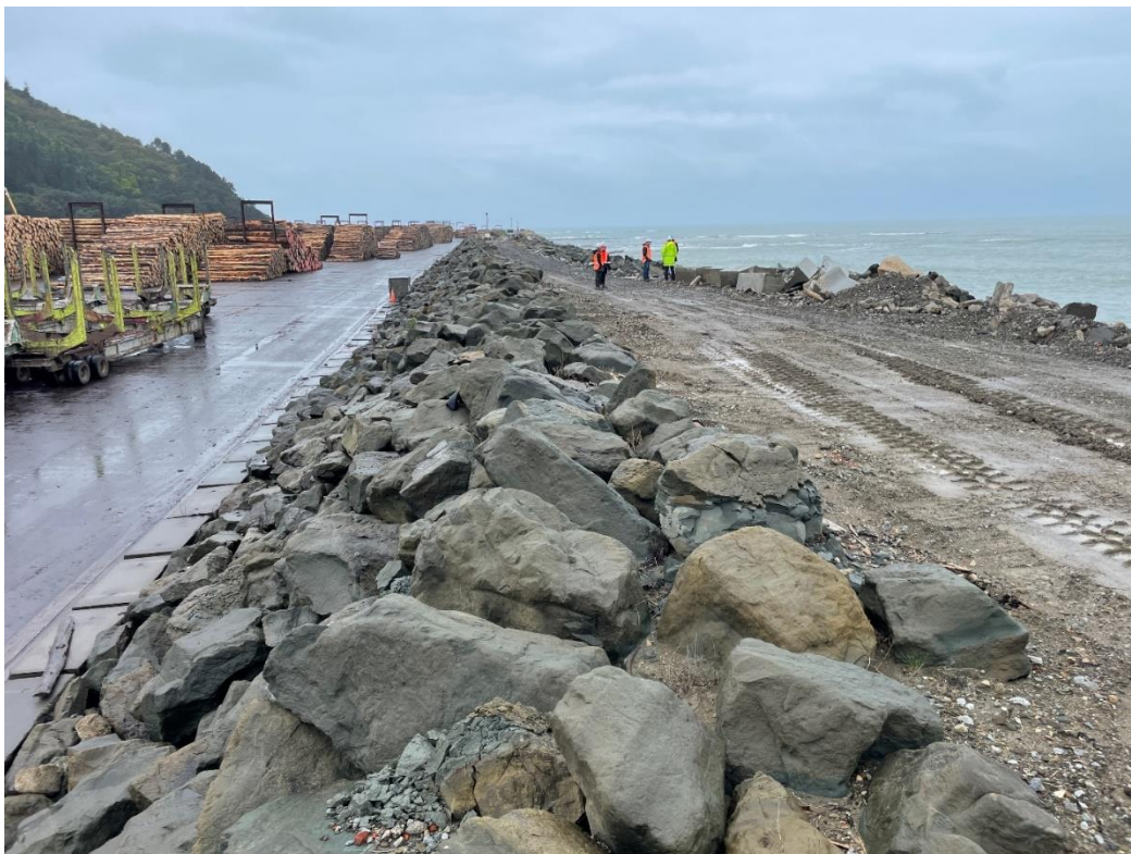
Figure 8: Inner riprap seawall that separates the logyard from the road and the outer seawall that will be deconstructed.
