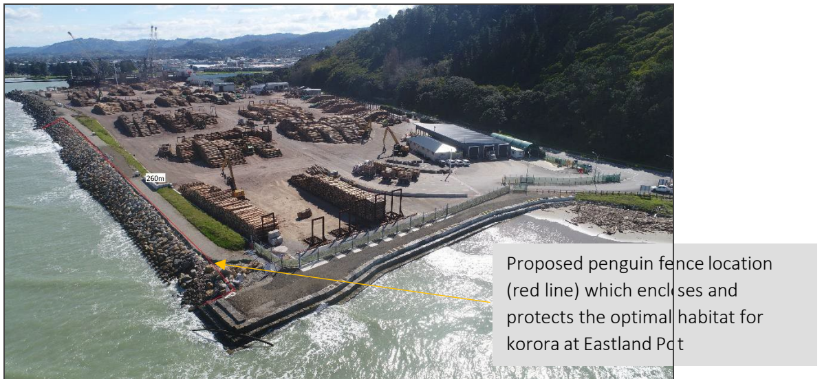
Fig 18: Aerial view of the Southern log yard revetment wall and proposed location of the penguin fence.
