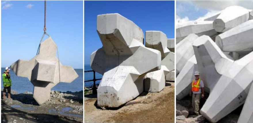
Figure 3-5 – Left – X-bloc® (4 m 3 /9.6 t, Port Oriel, Ireland). Centre – Accropode units (6.2 m 3 /14.9 t, Scarborough UK). Right – Core-loc® (15 m 3 /36 t, Kaunapau Harbor, Hawaii). (Reedjik & Muttray, 2009)
