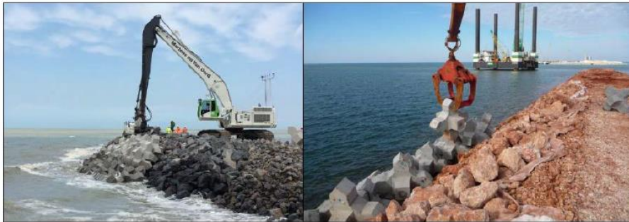
Figure 3-6 – Examples of typical random placement of X-bloc® units
