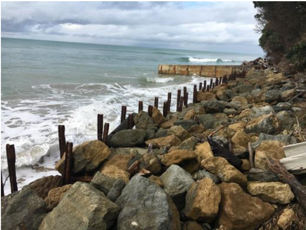
Figure 2: Existing sea wall from public access steps
