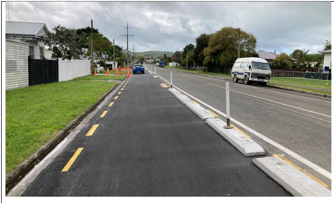
Figure 7 – Crawford Road, viewed looking east
