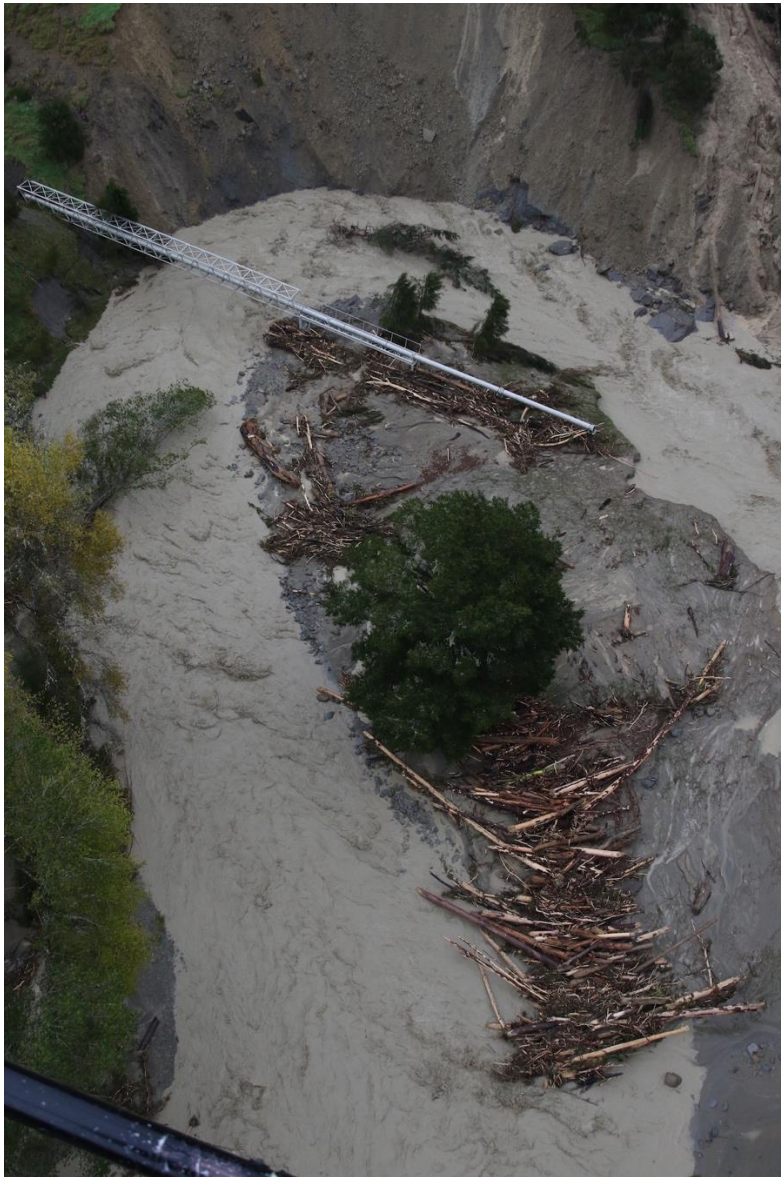
Figure 6 impacts on infrastructure
