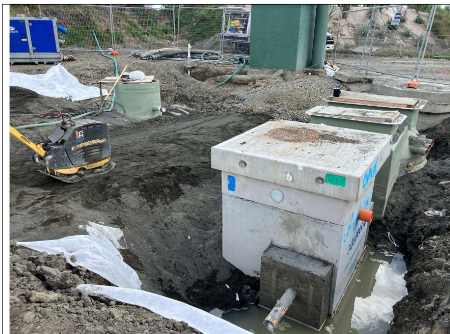
New Back Ormond Road Pump Station - early Dec 2023
