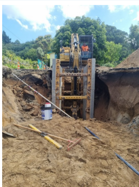
Douglas/ Frances Street stormwater pipe crossing looking north
