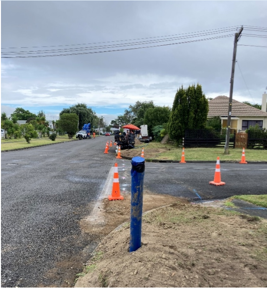
Redmond/Andrew streets intersection showing 125mm pipe crossing
