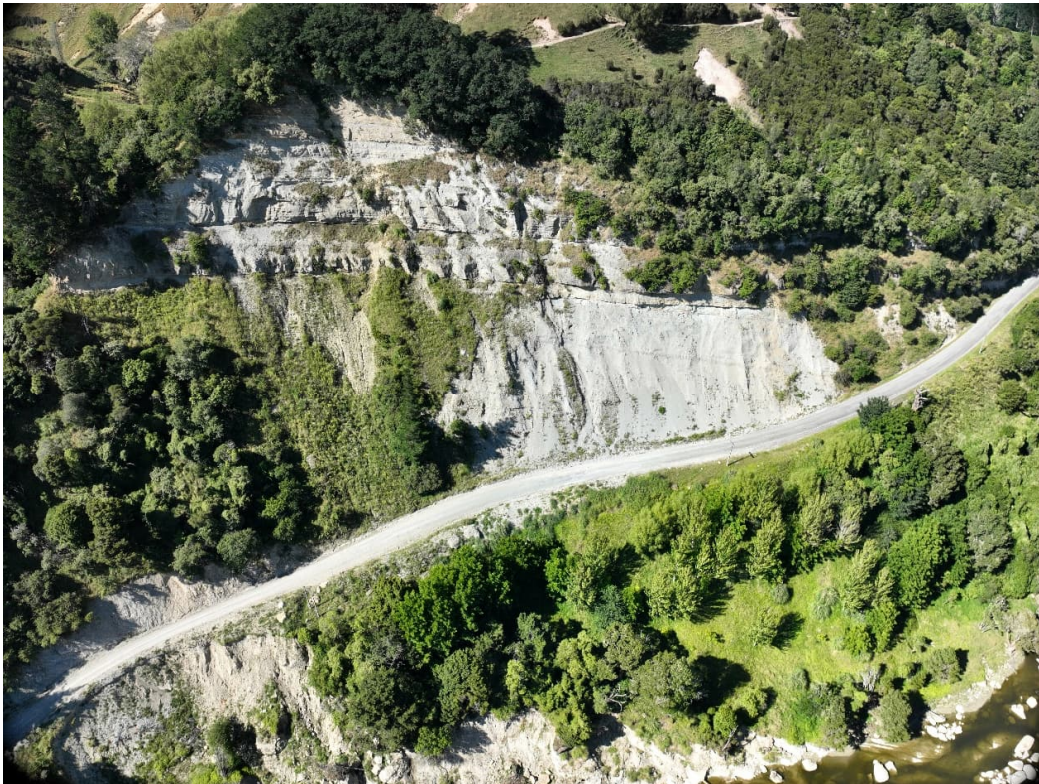
Figure 11: UAV to southwest of Bluff 3. Closer examination reveals large boulders that have reached the road or beyond in past events.
