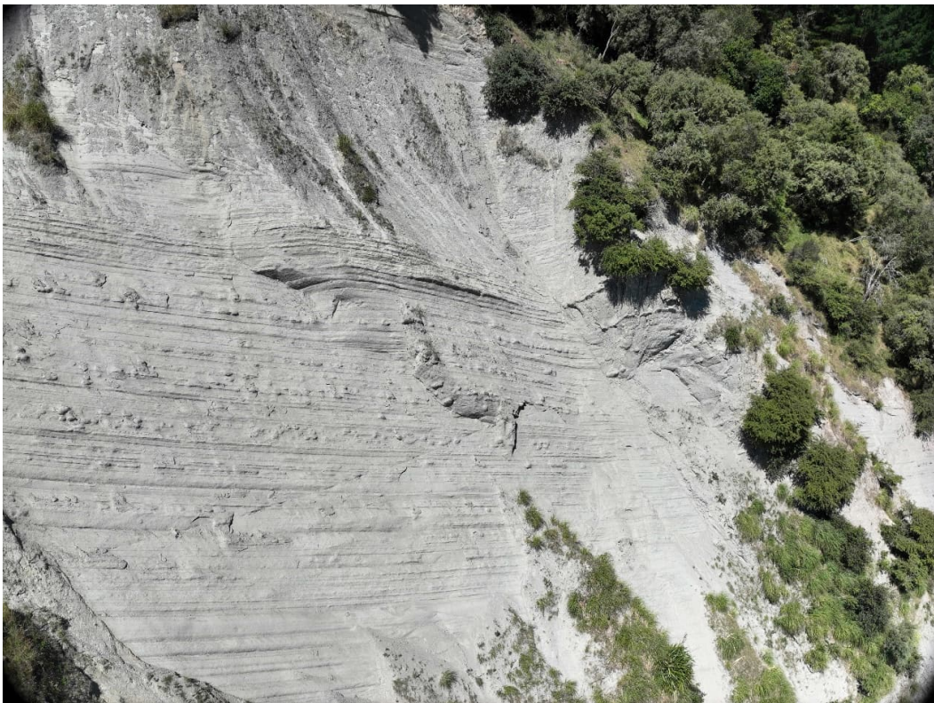
Figure 2: Oblique view to southwest of upper middle section of Bluff 1. Large blocks overhand areas where failure has already occurred, above a secondary defect.
