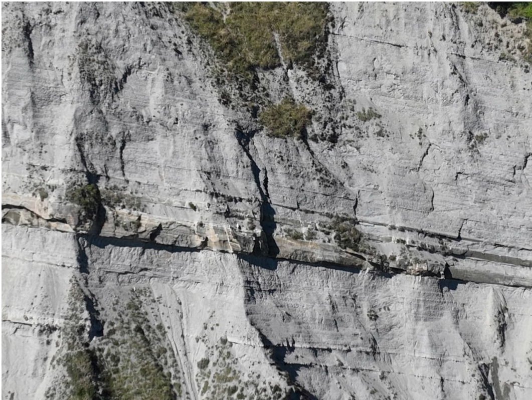
Figure 9: Overhanging sandstone bedding above more erodible mudstone in Bluff 2. Blocks fall from great height and are often channelled through the chutes into the roadway.
