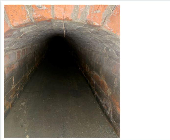
Childers Road / Disraeli Street brick stormwater channel
