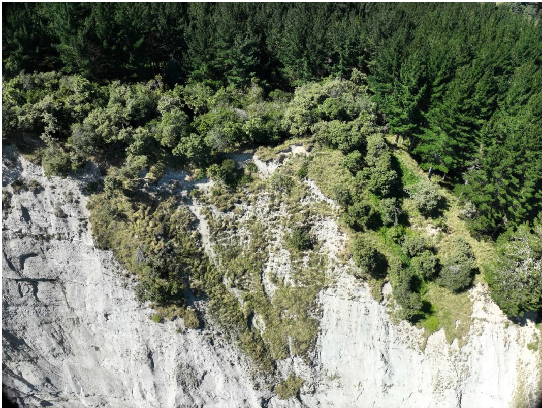
Figure 10: Displaced mass of residual soil and vegetation at the top (southwest) of Bluff 2. Future slide failure hazard.
