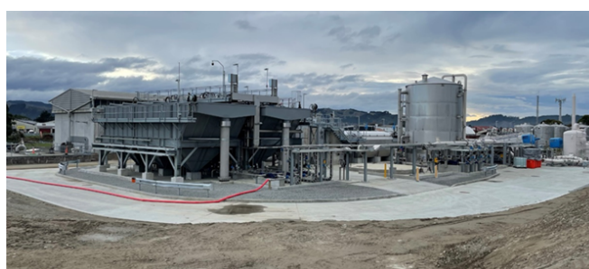
Wastewater Treatment Plant – Stage 2 Upgrade
