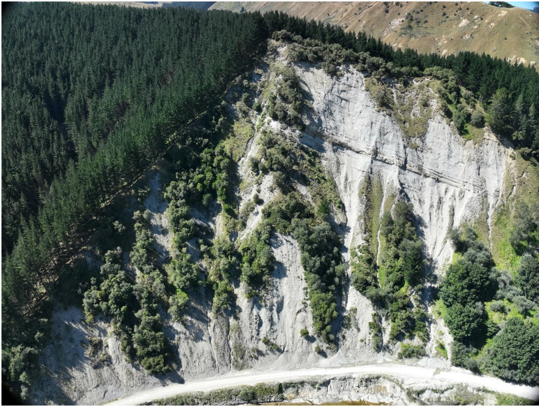
Figure 7: UAV view to south of Bluff 2. The channelised character of the slope is evident, with talus slopes and debris fans along the slope toe pushing into the roadway. Water flow was minimal after an extended period of dry weather. The debris fans have blocked the narrow drain/ditch which pushes stormwater flow over the road.
