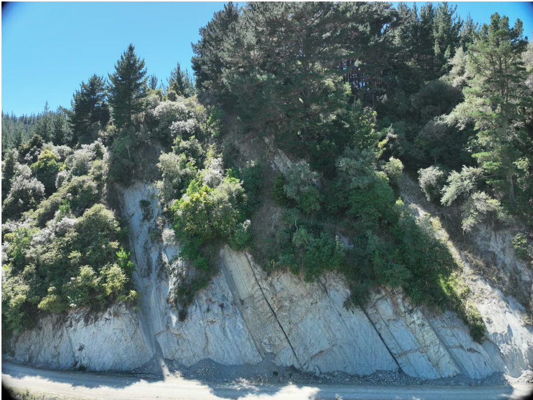
Figure 5: Contractor cut face before Bluff 1 between 34.3 and 34.6.
