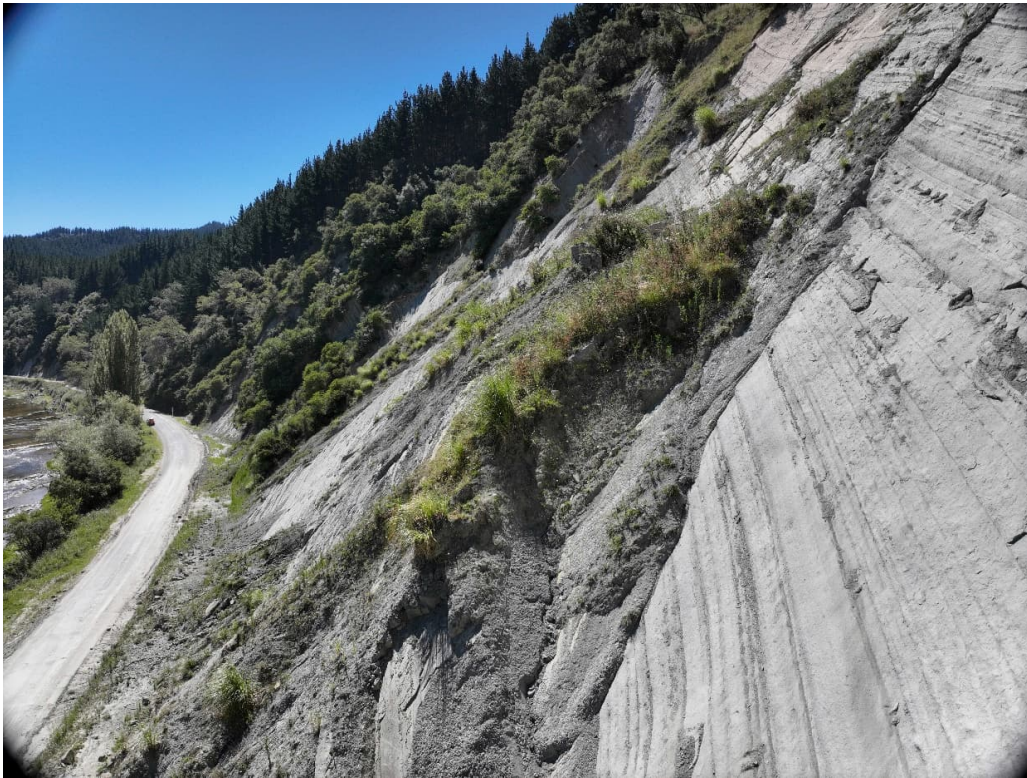
Figure 3: UAV view to east of Bluff 1 along planar (structural defect-controlled face). Perched blocks of weathered rock/soil and vegetation are evident, intersected by the pervasive defect. A remnant of an earth bund and accumulated sediment are evident at the slope toe.
