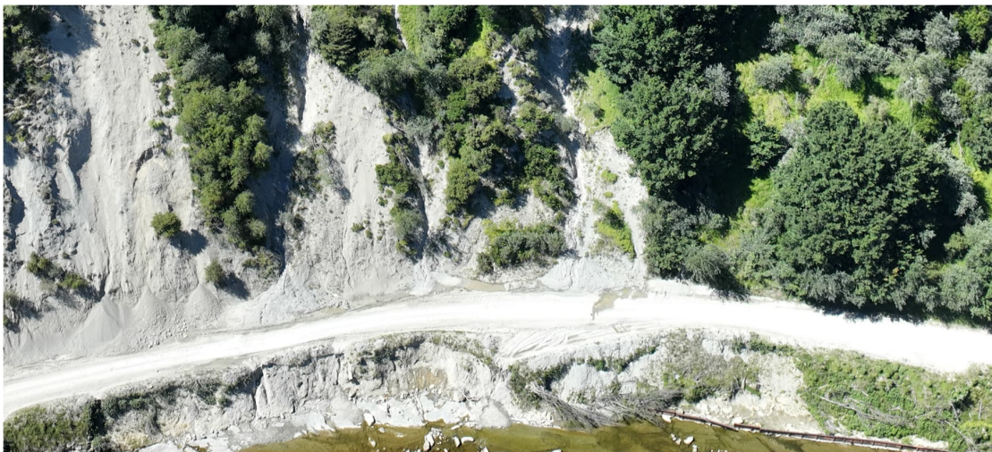
Figure 8: Dropouts along mid-section of Bluff 2. A culvert is visible in one of the dropouts, showing the extent of bank loss. Further west is a damaged section of retaining wall.
