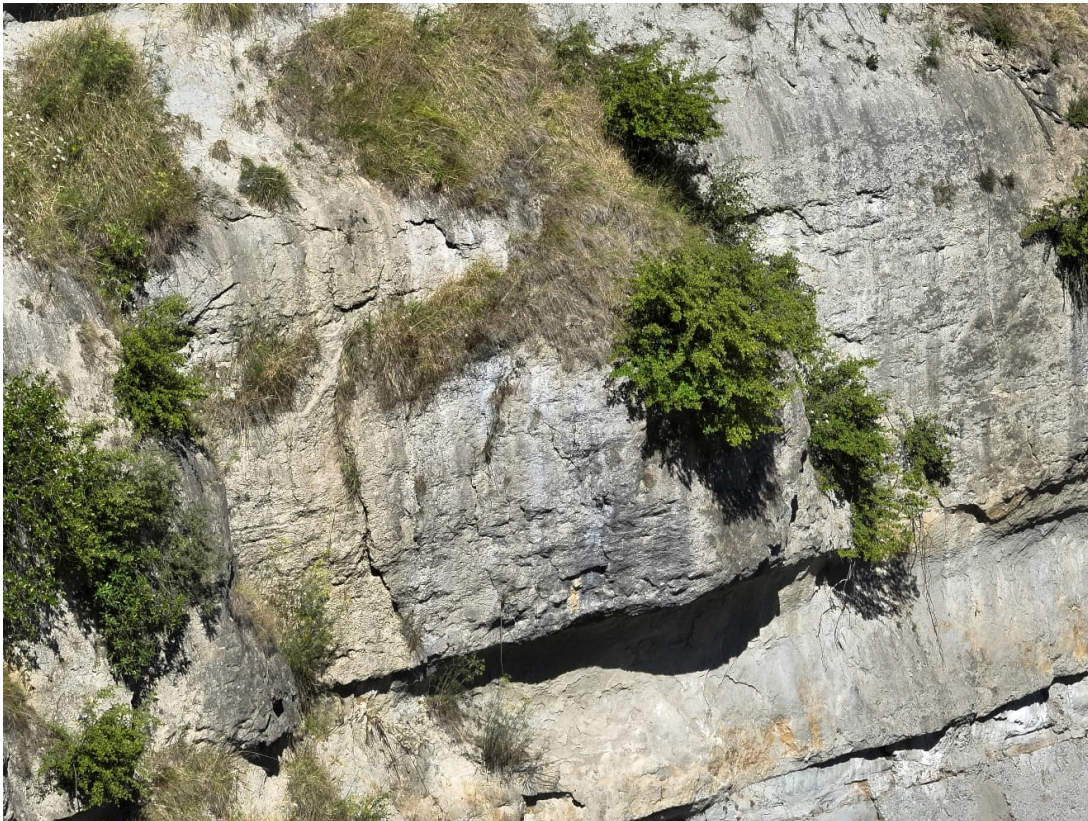
Figure 14: Close up, viewed to west, of dilated cracks in large block of overhanging sandstone.
