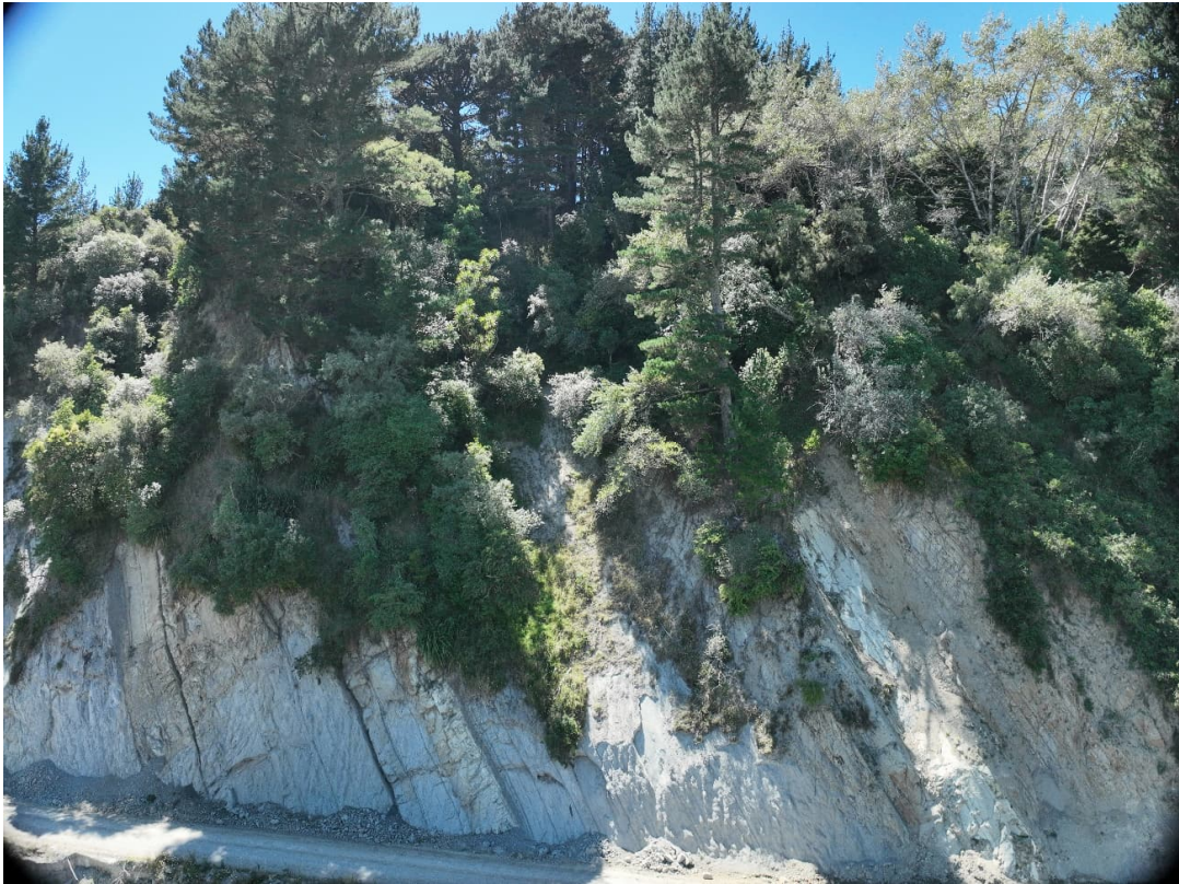
Figure 6: Contractor cut face before Bluff 1 between 34.3 and 34.6.
