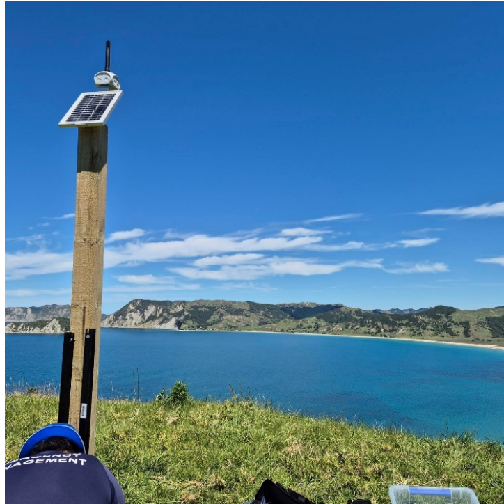
Marcus Tibble (TEMO) Solar Repeater Installation at Anaura Bay
