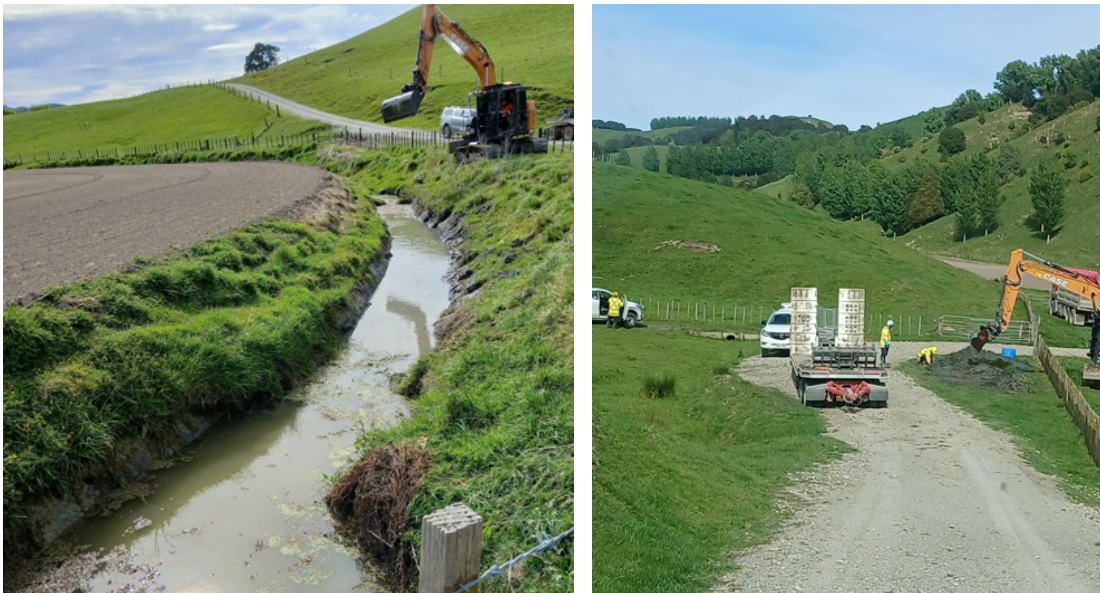
'Contour' Drain Regrades & Eel relocation
