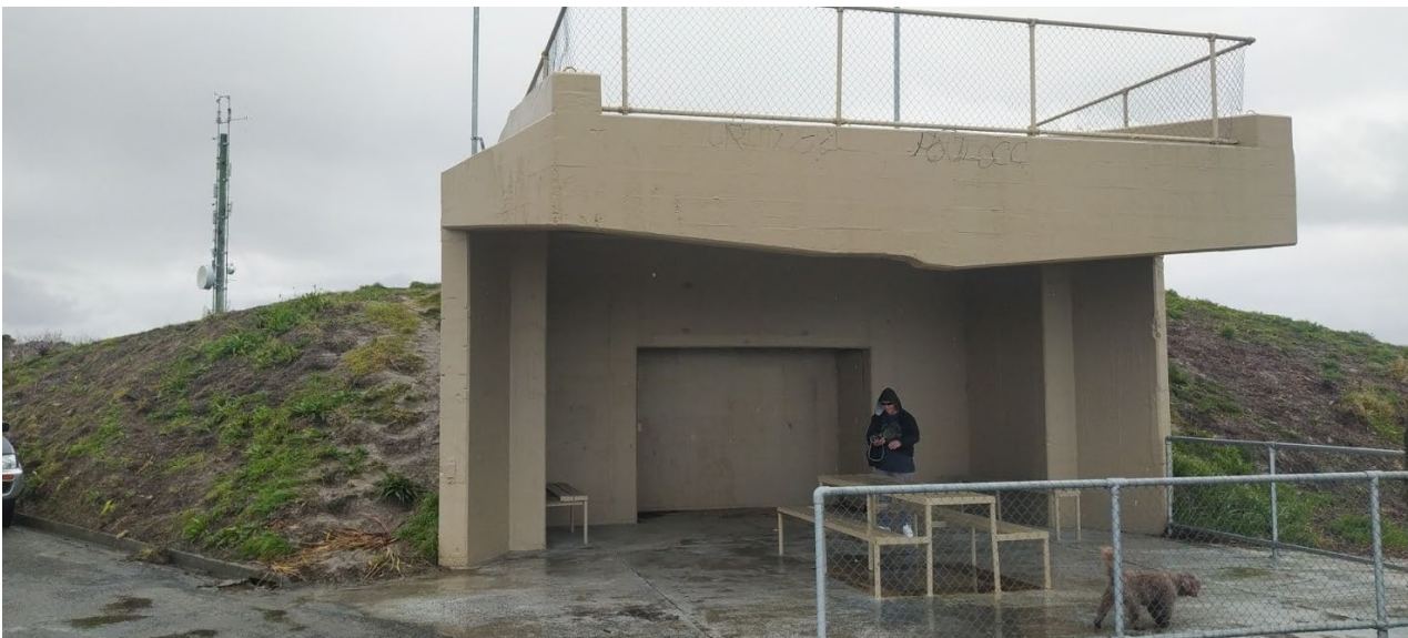
Figure 11: Photo of Existing WW2 Gun Emplacement Structure (Source: 4Sight Consulting Limited)
